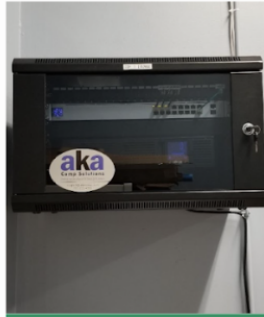
IDF RACK MOUNTS SECURED INSTALLS
