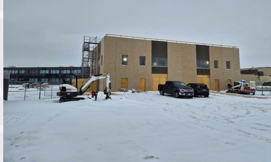
Auto Shop Addition (Storm Shelter)
