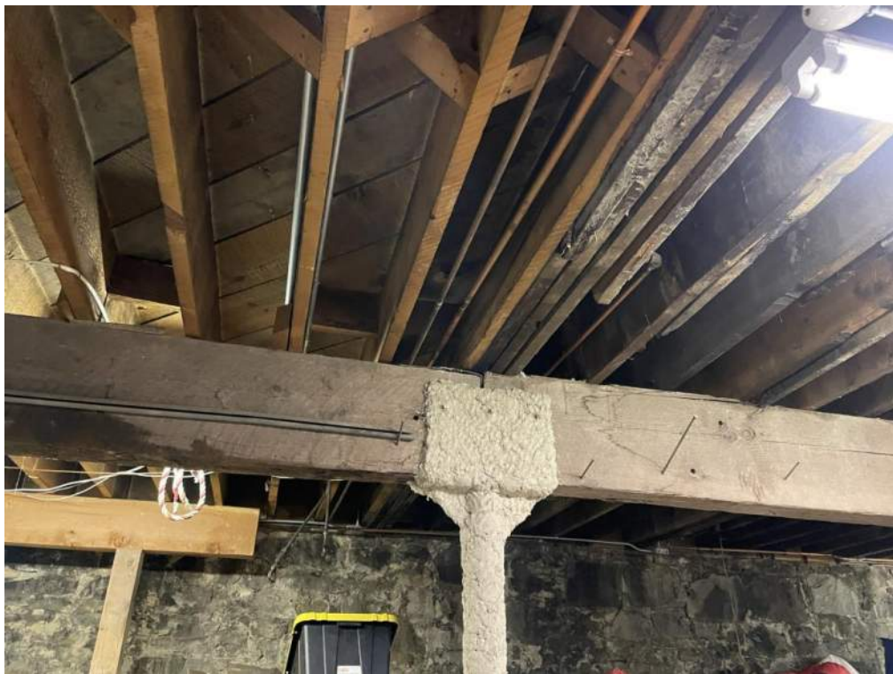
Figure 14- Upgraded column in basement. Note stone basement wall in background.
