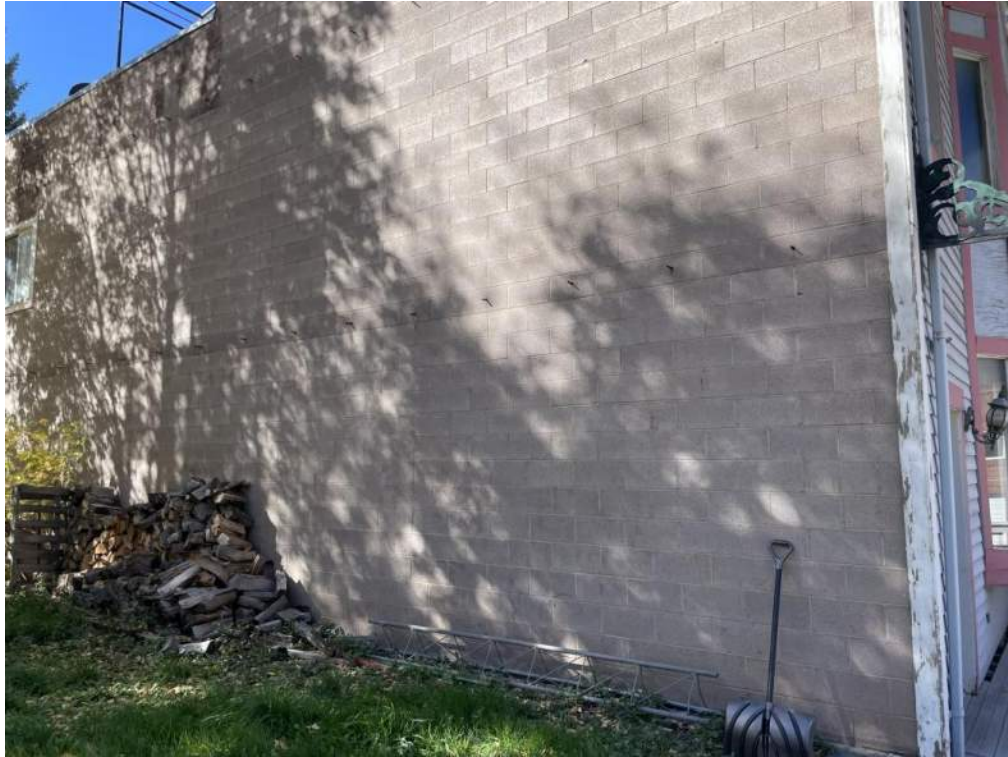
Figure 11- Exterior load-bearing CMU wall.
