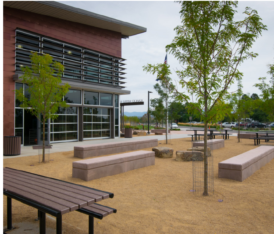
Crusher fines plaza surface
