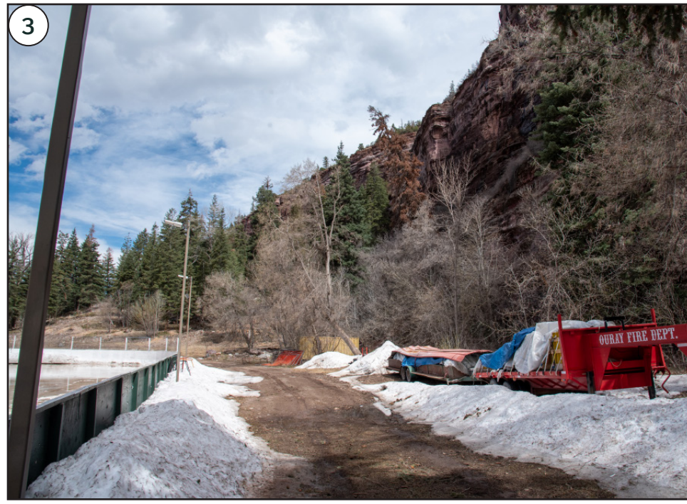
3 Storage Area Analysis: Relocate or screen storage area.
