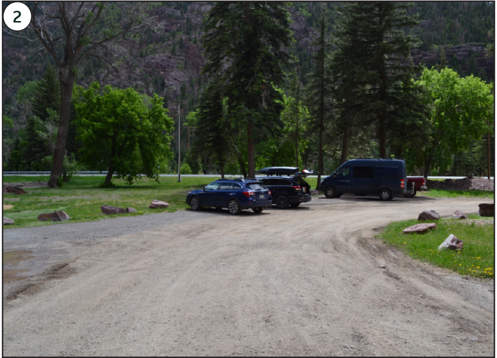
2 Parking Analysis: Reduce number of roads and consolidate parking to increase square footage of usable park spaces and improve pedestrian safety.
