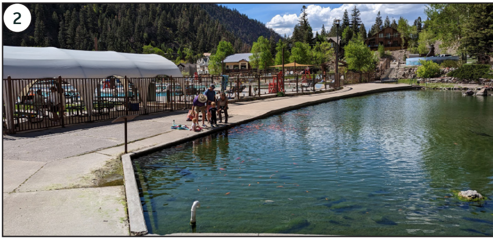
2 Fish Pond Analysis: Need to improve concrete at fish pond.
