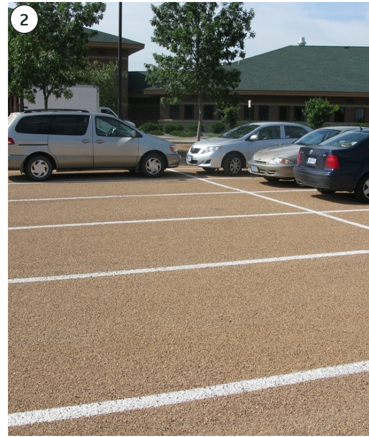
Delineate parking areas by temporary striping
