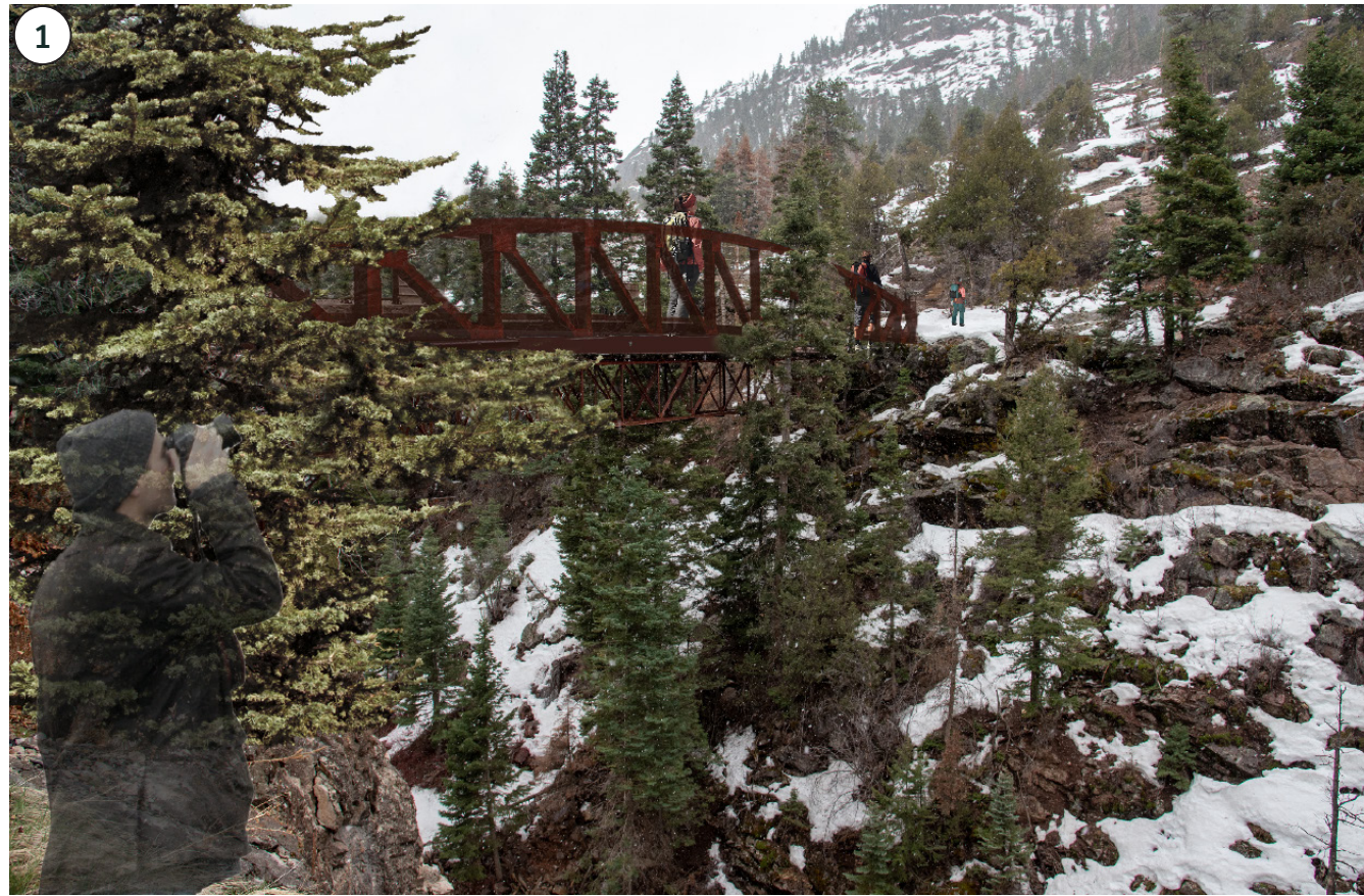
New pedestrian bridge for trail access to Box Cañon
