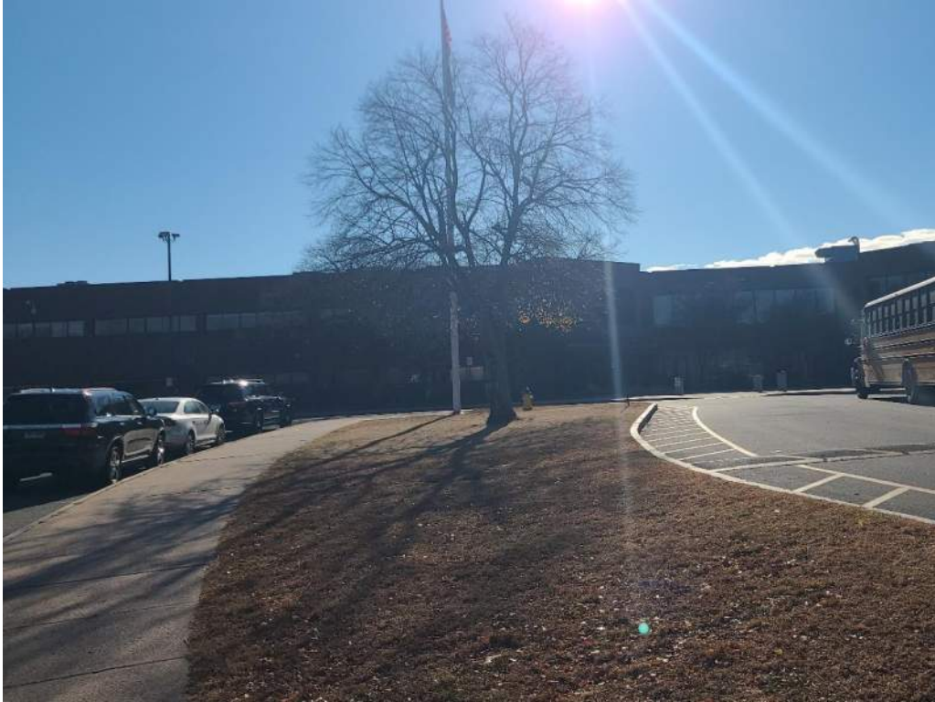
Photograph 1 – Overall View of School
