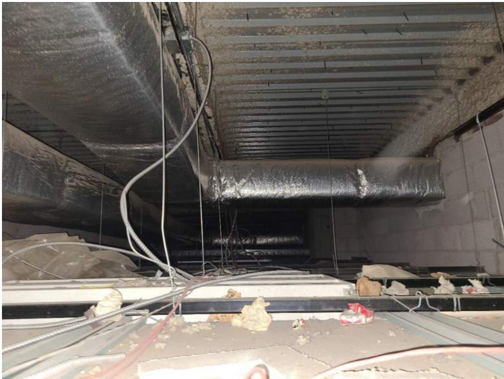
Photograph 6 – Overall View of Roof Framing in Original Wing
