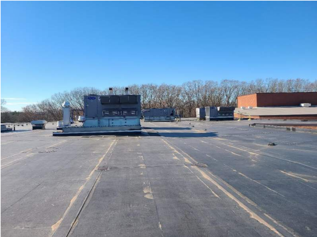
Photograph 12 – Overall View of Roofing
