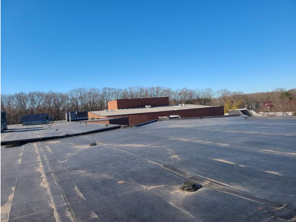
Photograph 11 – Overall View of Roofing
