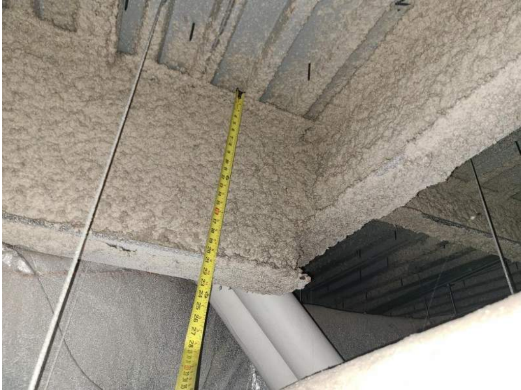
Photograph 9 – Overall View of Library Roof Framing
