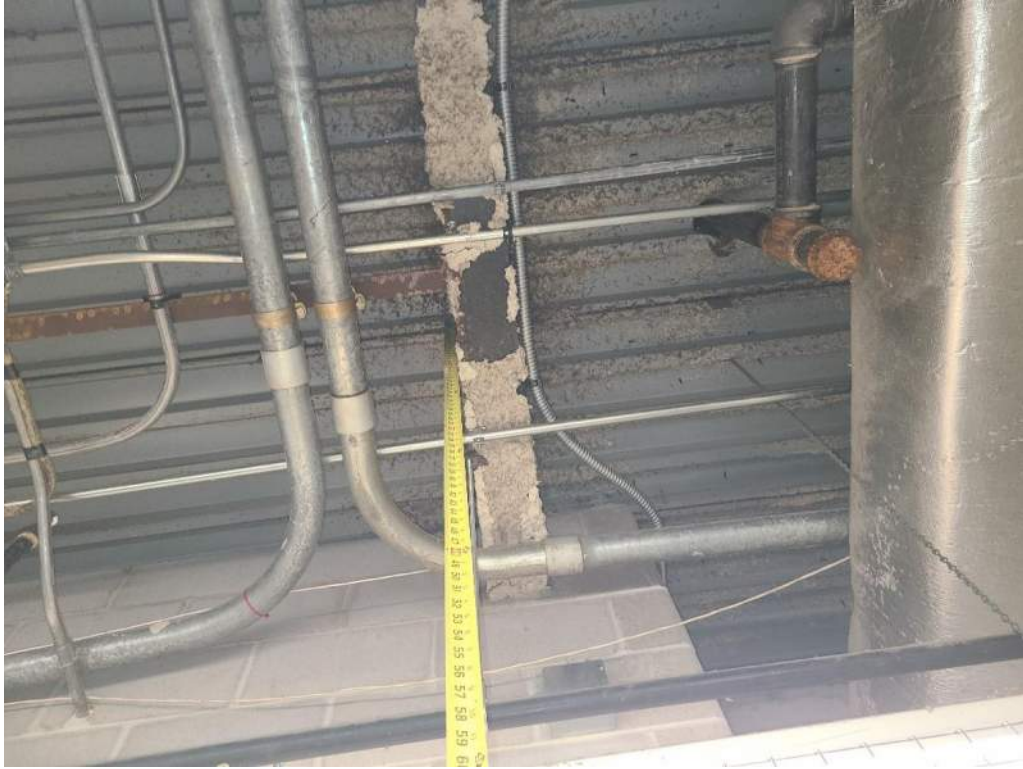
Photograph 5 – Overall View of Roof Framing in Original Wing
