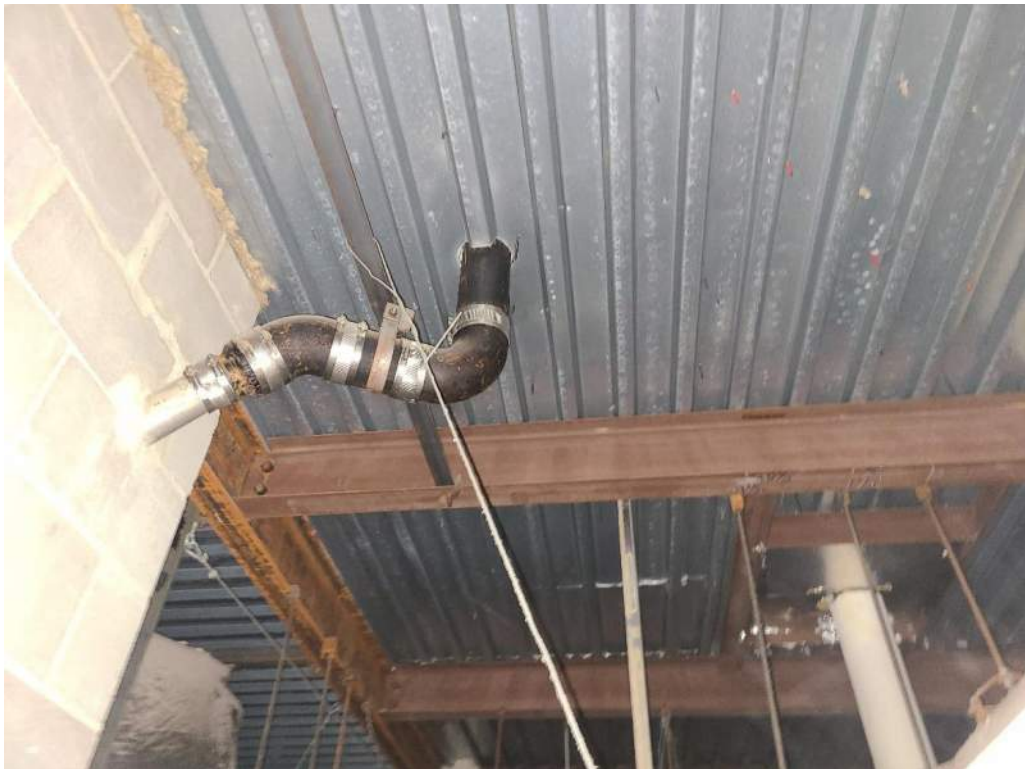
Photograph 4 – Overall View of Roof Framing in Freshman Wing
