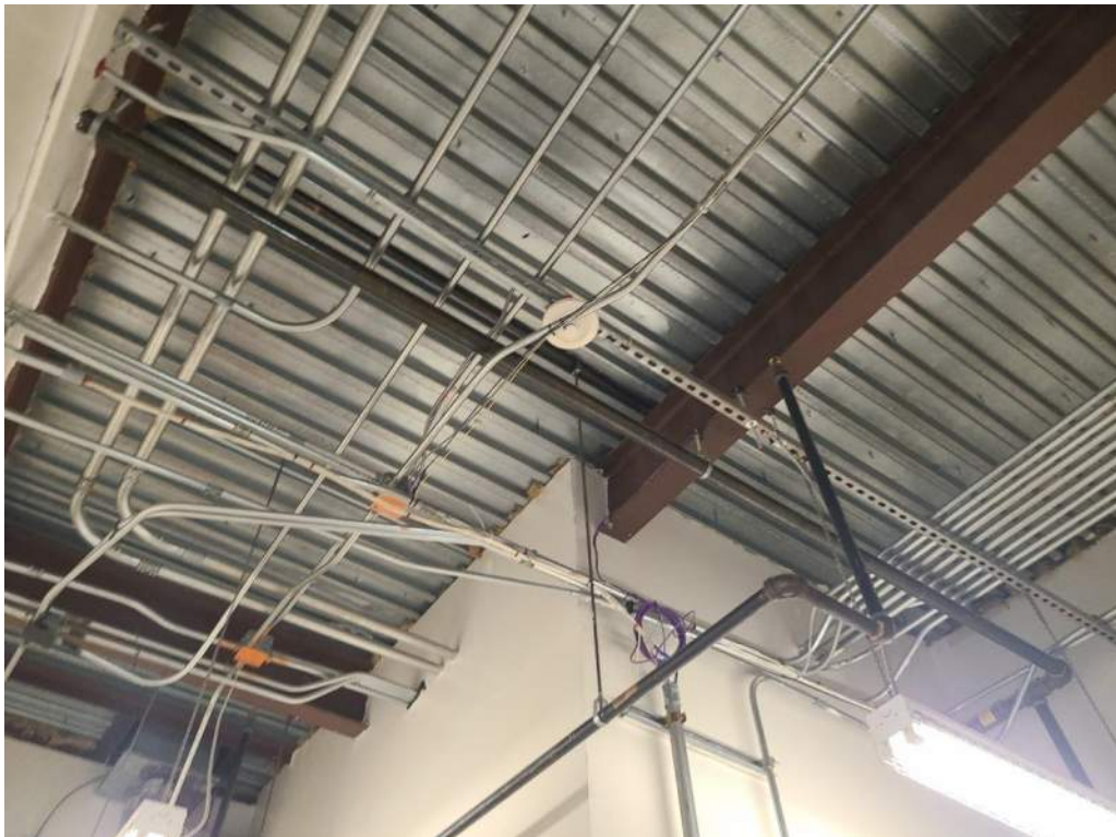
Photograph 2 – Overall View of Roof Framing in Freshman Wing
