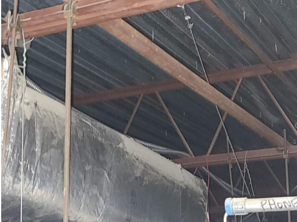
Photograph 3 – Overall View of Roof Framing in Freshman Wing
