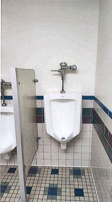
Wesley boys bathroom repair ^
