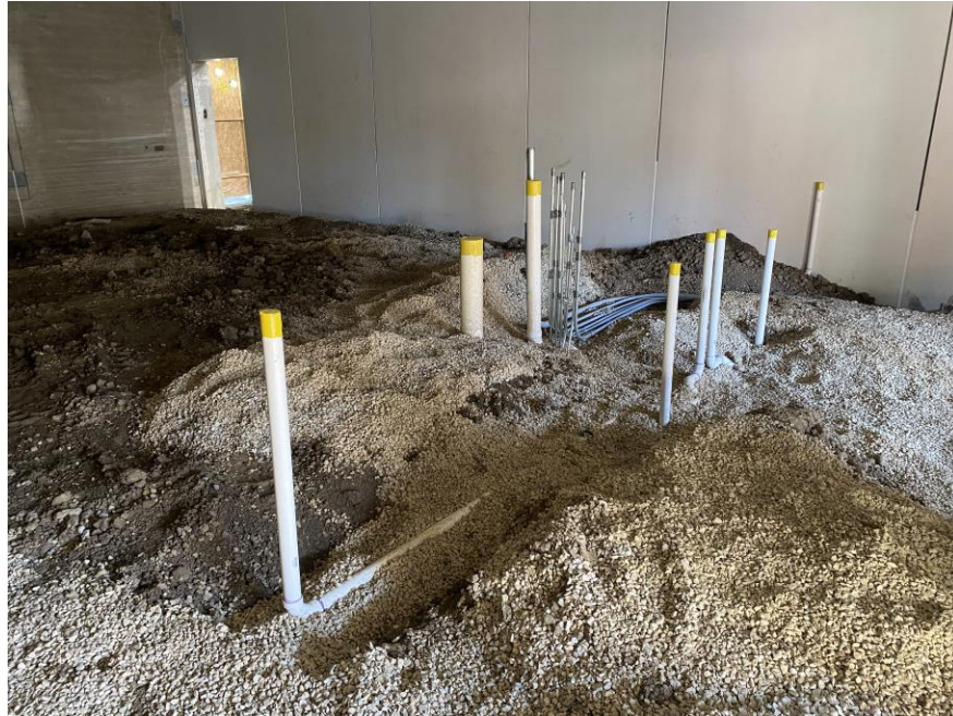
Underground Plumbing at New Gym Locker Rooms
