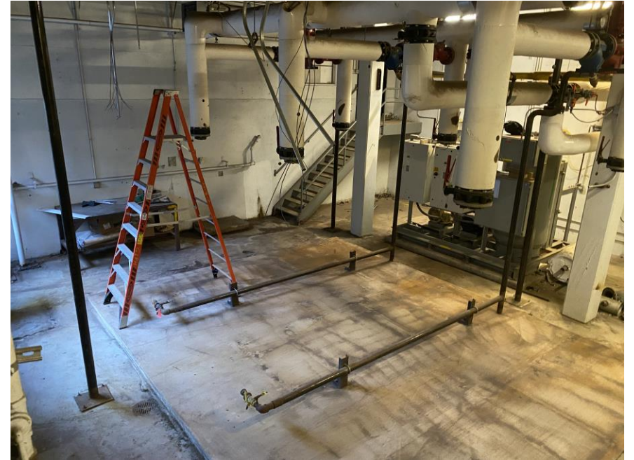
Boiler Demolition Completed
