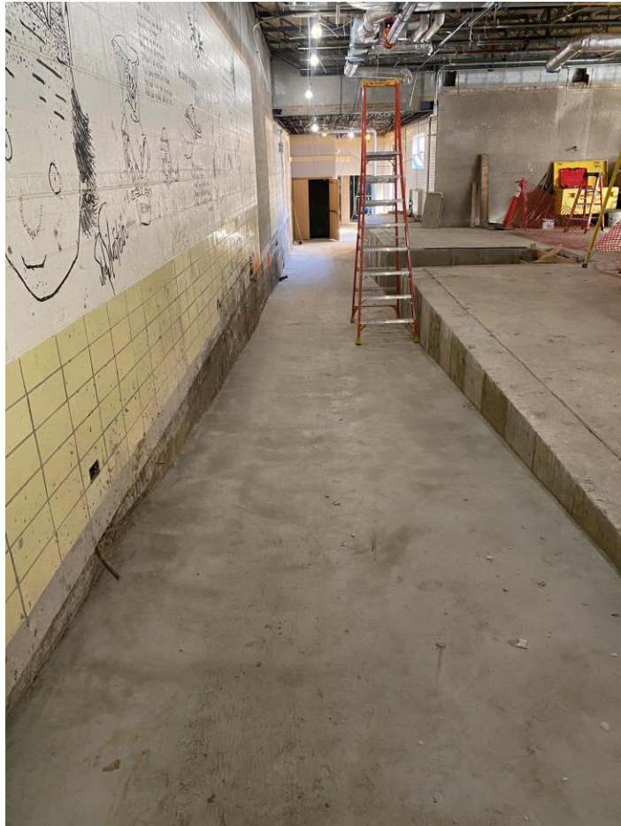
New East Side Ramp for ADA at Music Wing
