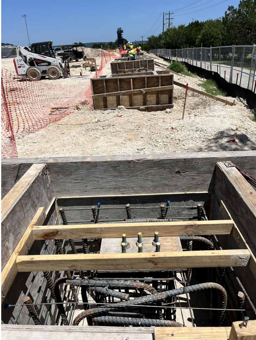
Photo: Piers at Multipurpose Covered
