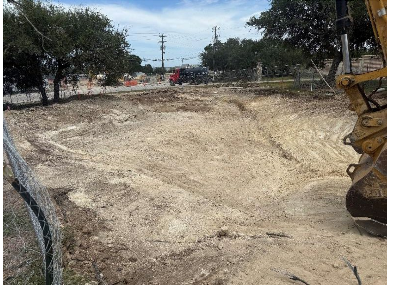
Photo: WHS Detention Pond
