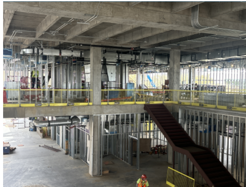
Overhead mechanical, electrical and plumbing- Lobby
