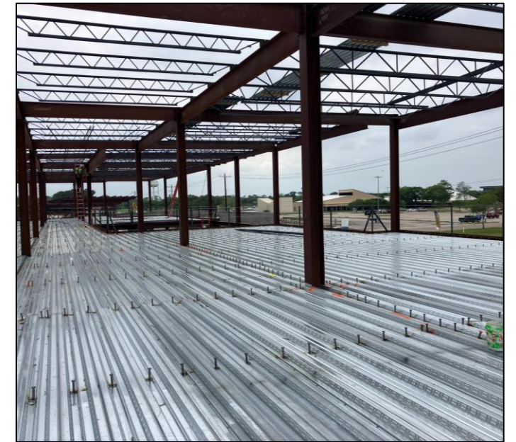
Metal deck, 2 nd floor, Area A
