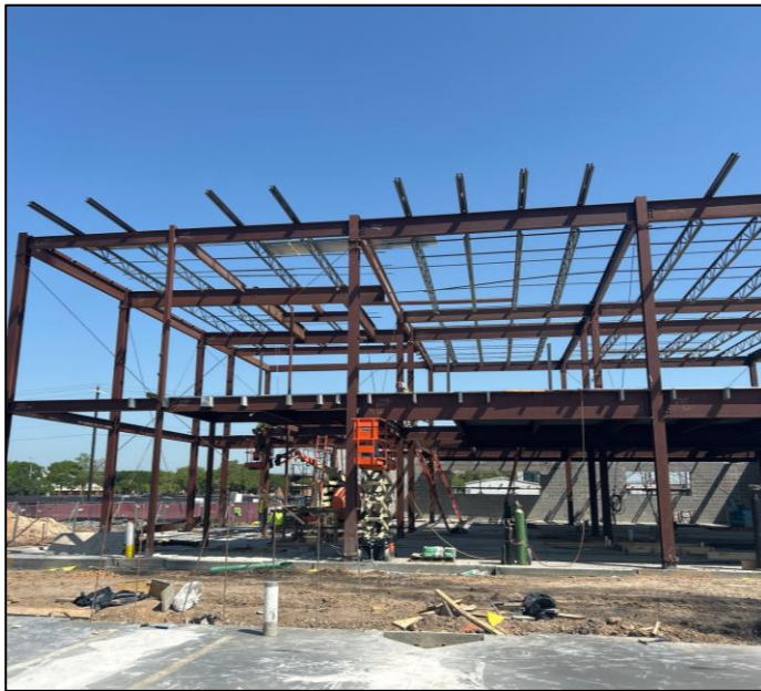
Structural steel erection
