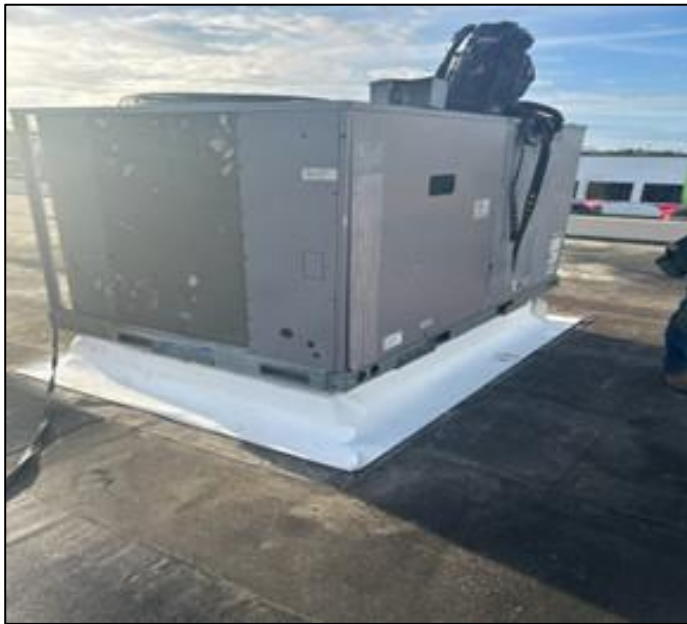
New Roofing Welding Building
