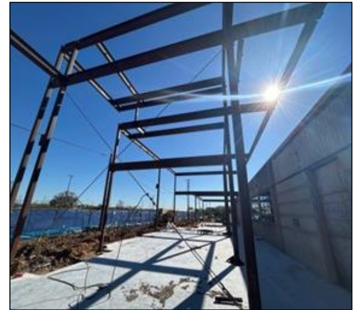
Structural Steel In Progress
