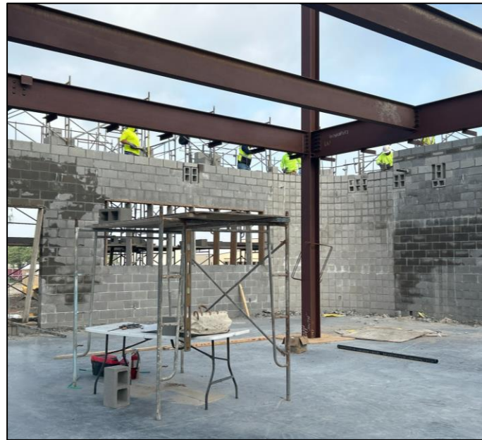
CMU wall, Area A
