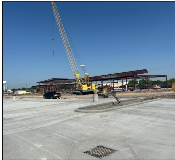
Concrete at parking lot
