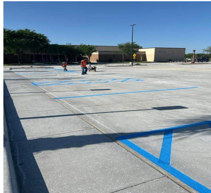
Lot B Striping in progress
