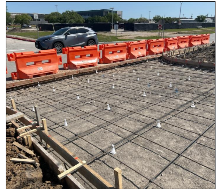
Prep for concrete pour, west driveway entrance
