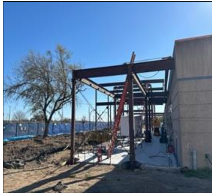
Welding Addition Structural Steel Installation
