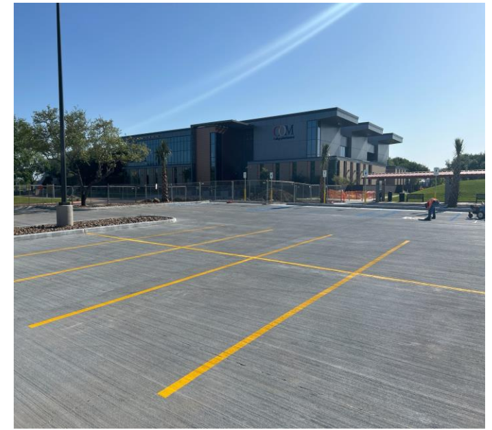
Lighting – Parking Lot B
