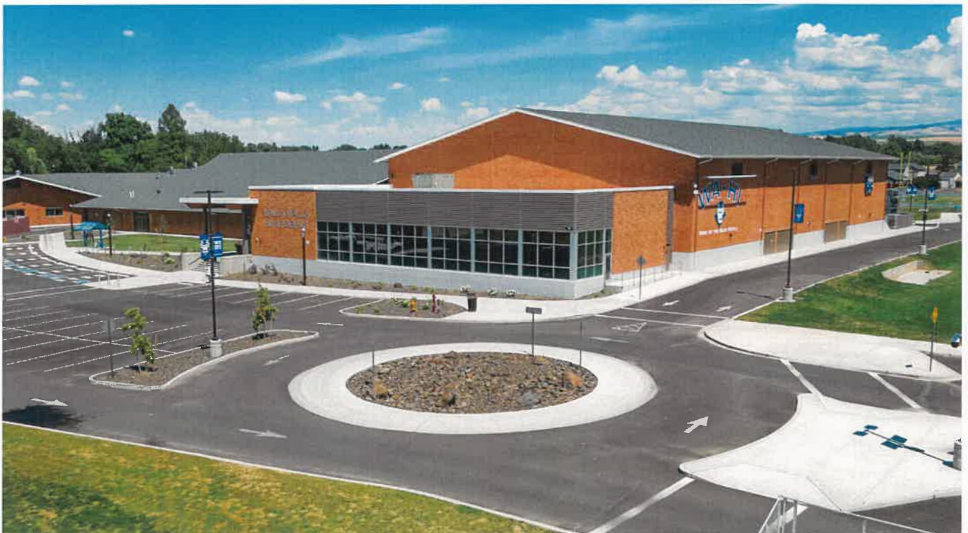
COORDINATOR FOR REPAIRS OF PRIEST RIVER JUNIOR HIGH
