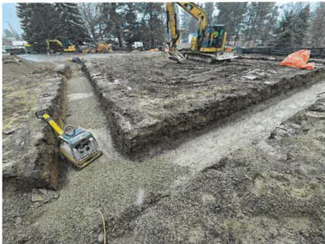
Prepping for Footings & Foundation Walls
