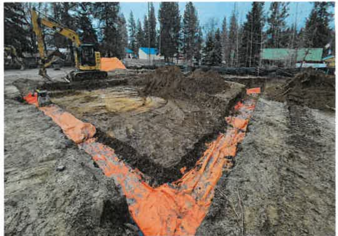
Prepping for Footings & Foundation Walls
