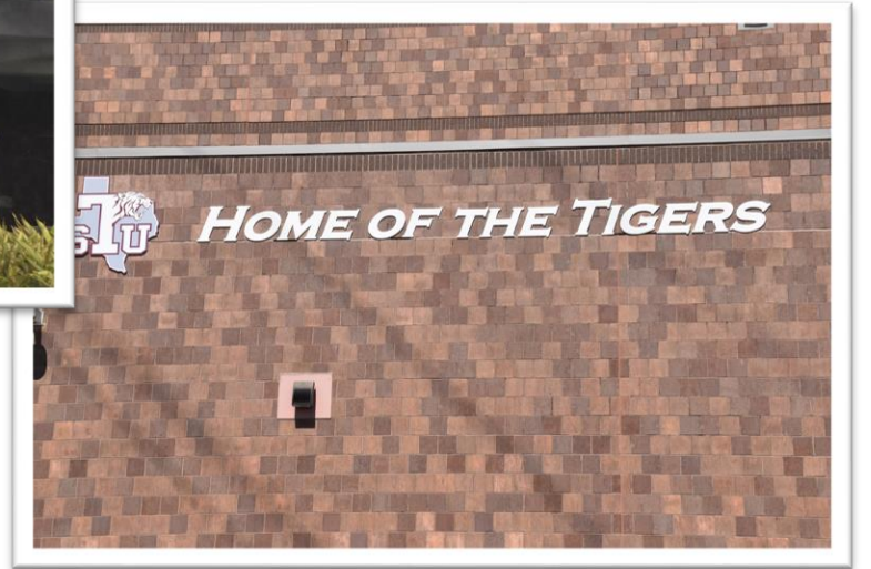
Backside facing the Rec Center and the Fieldhouse
