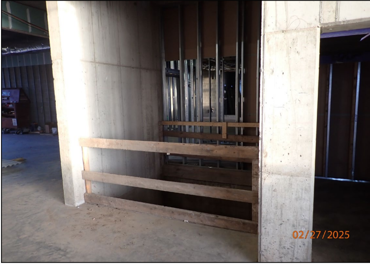
13 1st Fl., Elevator shaft
