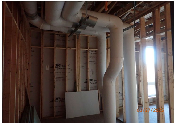
Roof piping installation underway
