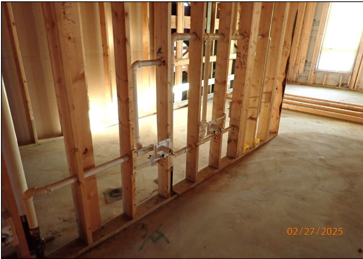
17 2nd Fl., Bathroom plumbing rough-in
