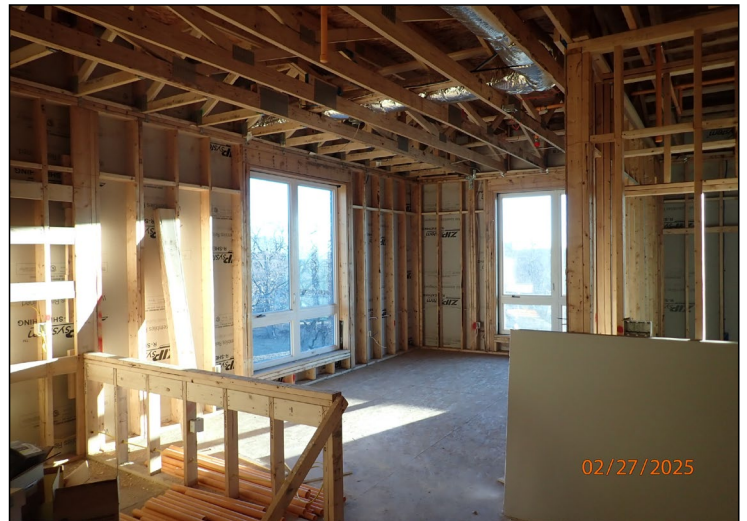
Unit, MEP underway
