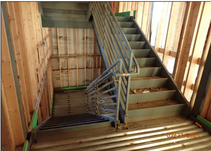
18 3rd Fl., Stairwell
