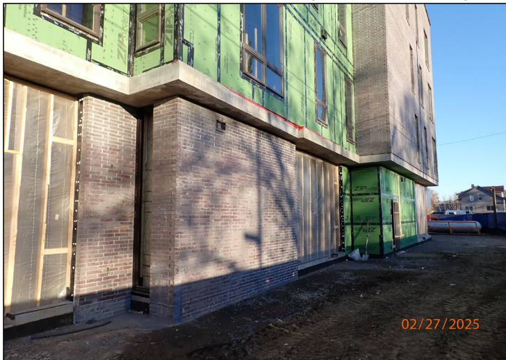
9 East & West sides, Masonry brick underway
