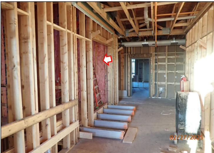
23 4th Fl., Elevator shaft, Insulation started
