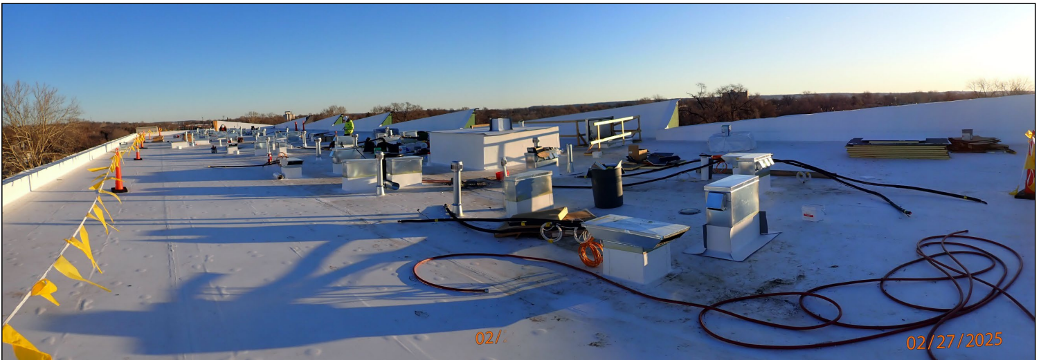
24 Roof-top, HVAC installation underway
