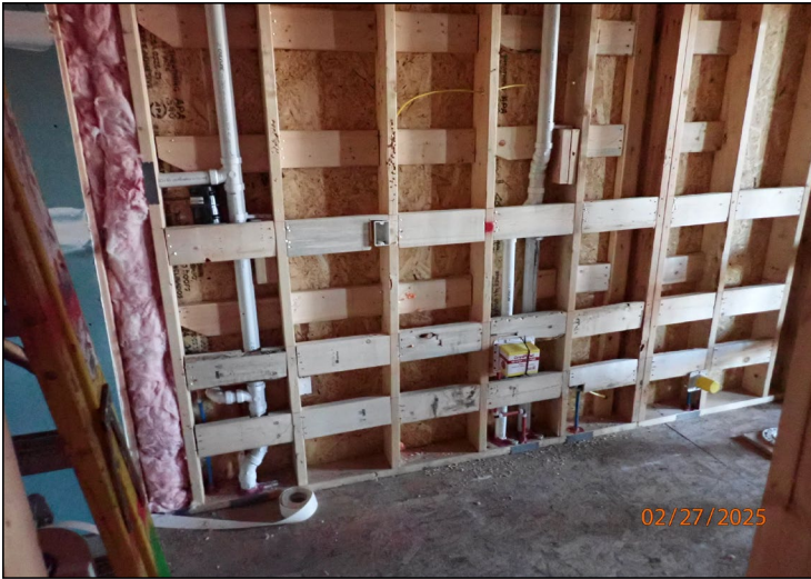
22 4th Fl., Bathroom plumbing rough-in
