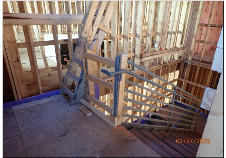
4th Fl., Stairwell
