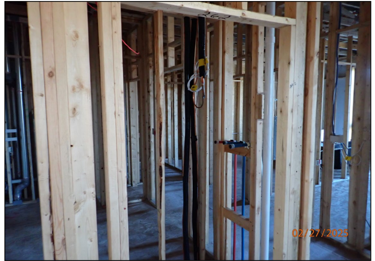
Water heater closet piping installation underway
