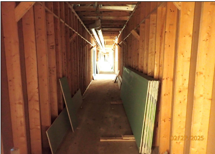
24 4th Fl., Corridor & Drywall materials
