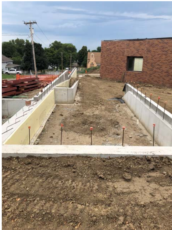
Entry tower and ramp foundation walls
