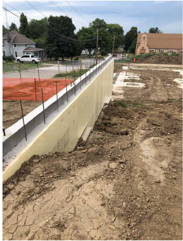
Foundation wall insulation on west wall
