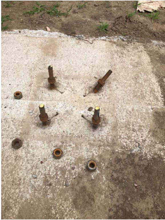
Try to straighten anchor bolt. If bolt breaks consult structural engineer for solution.
