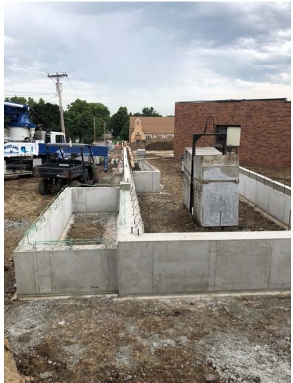
Structural stoop and tower entry foundations
