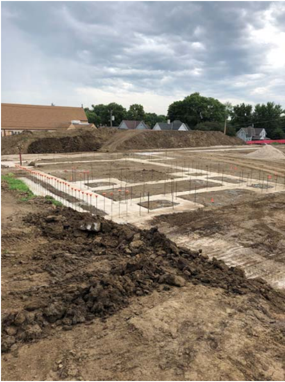
Footings for locker rooms
