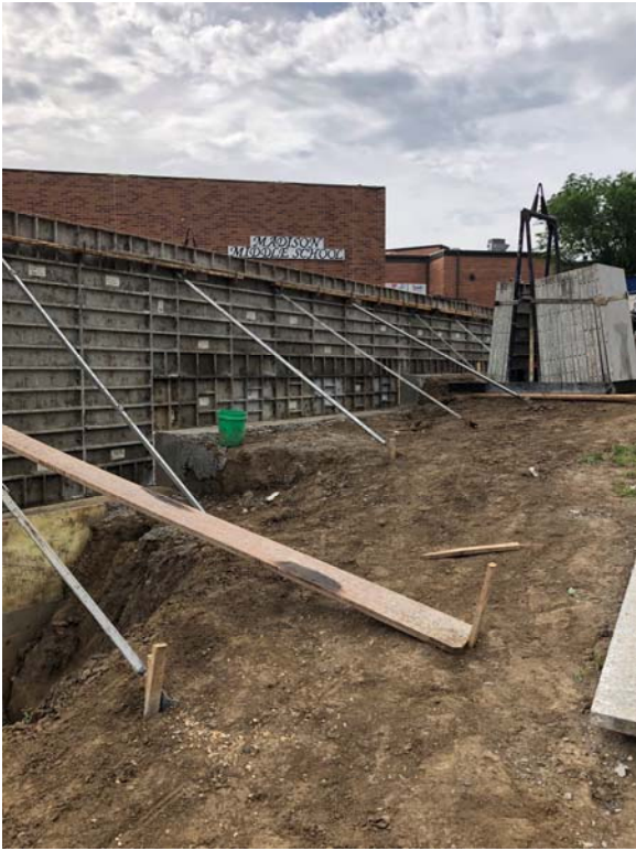
East wall footings and foundation walls
