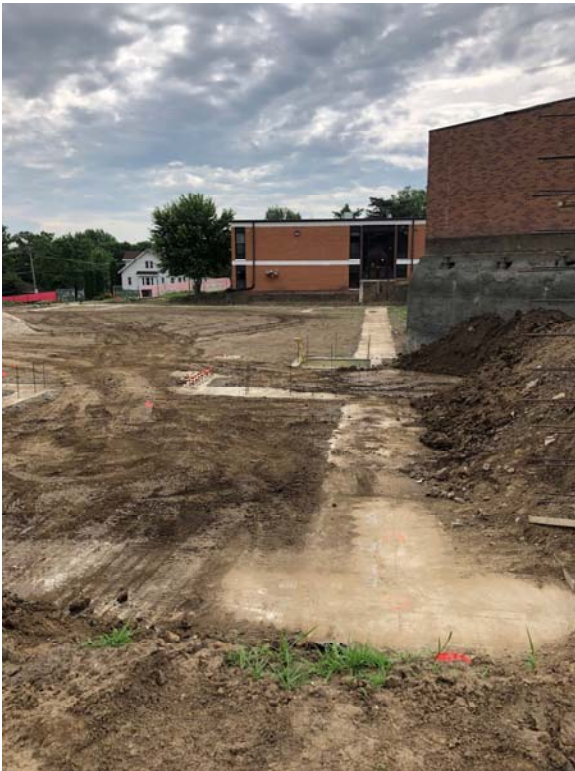
Footings south wall of Gymnasium
