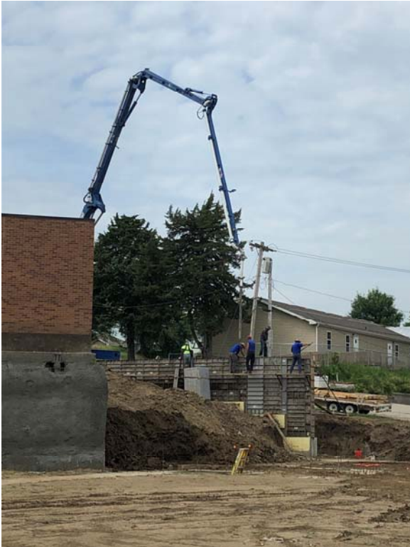
Concrete placement east foundation wall
