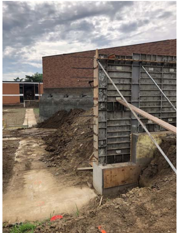
West wall footings and foundation wall at public restrooms
