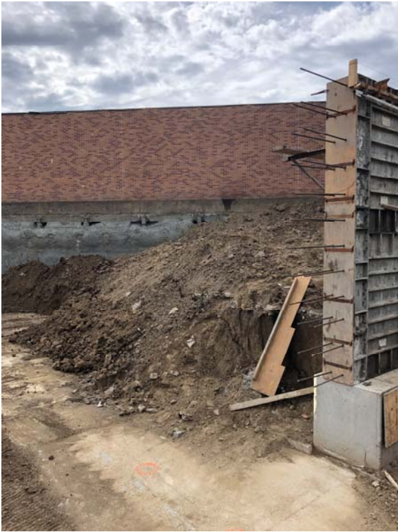
East foundation wall reinforcing steel
