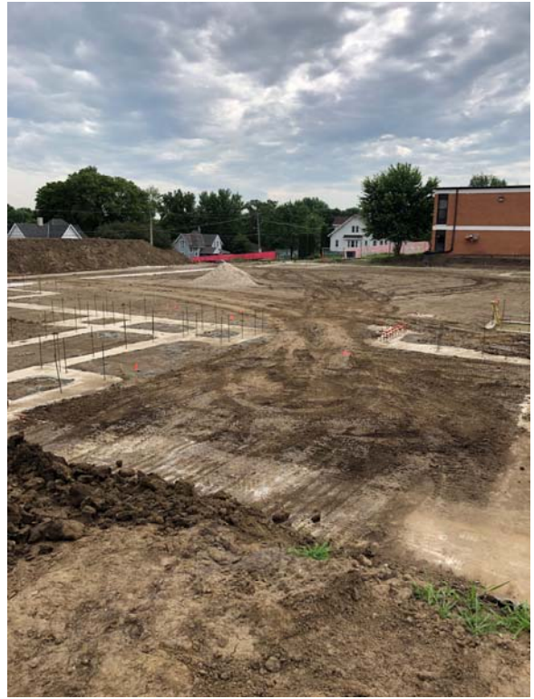
Locker rooms/gymnasium footings
