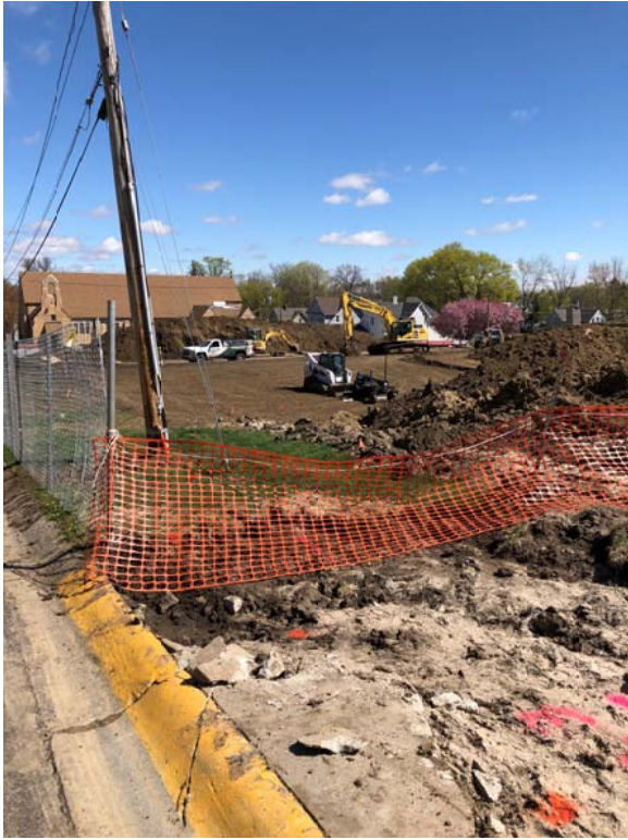
Gymnasium site looking North
