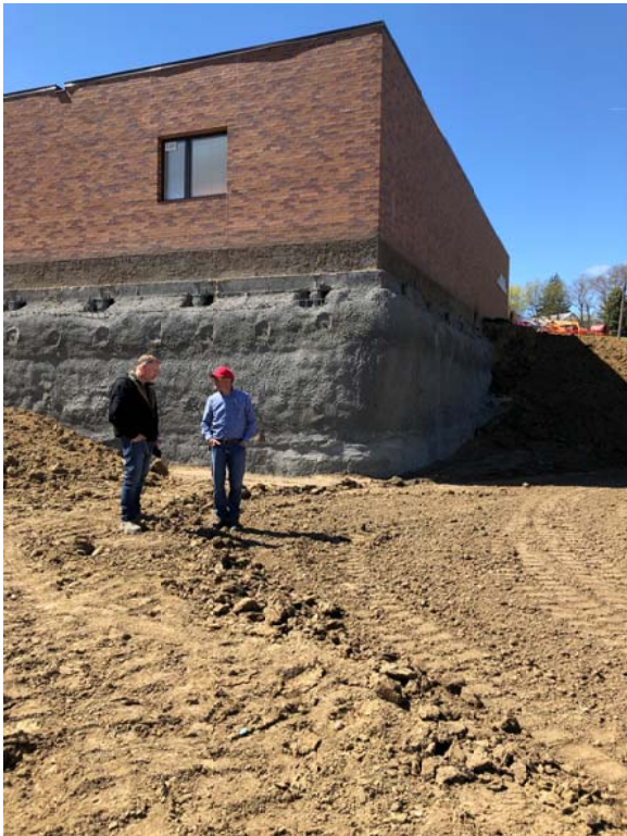
Underpinning of Middle School wing
