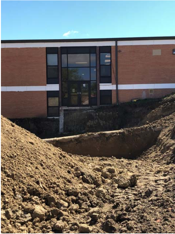
Stoop removal at North building
