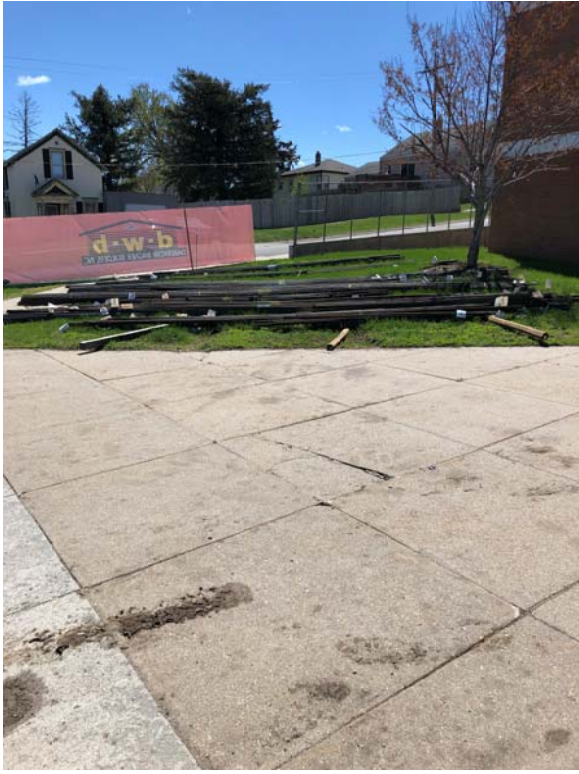
Stored reinforcing materials for gymnasium footings
