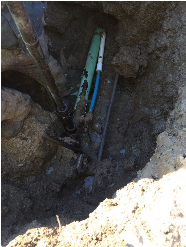
EXISTING YARD HYDRANT PIPING AT VALVE
