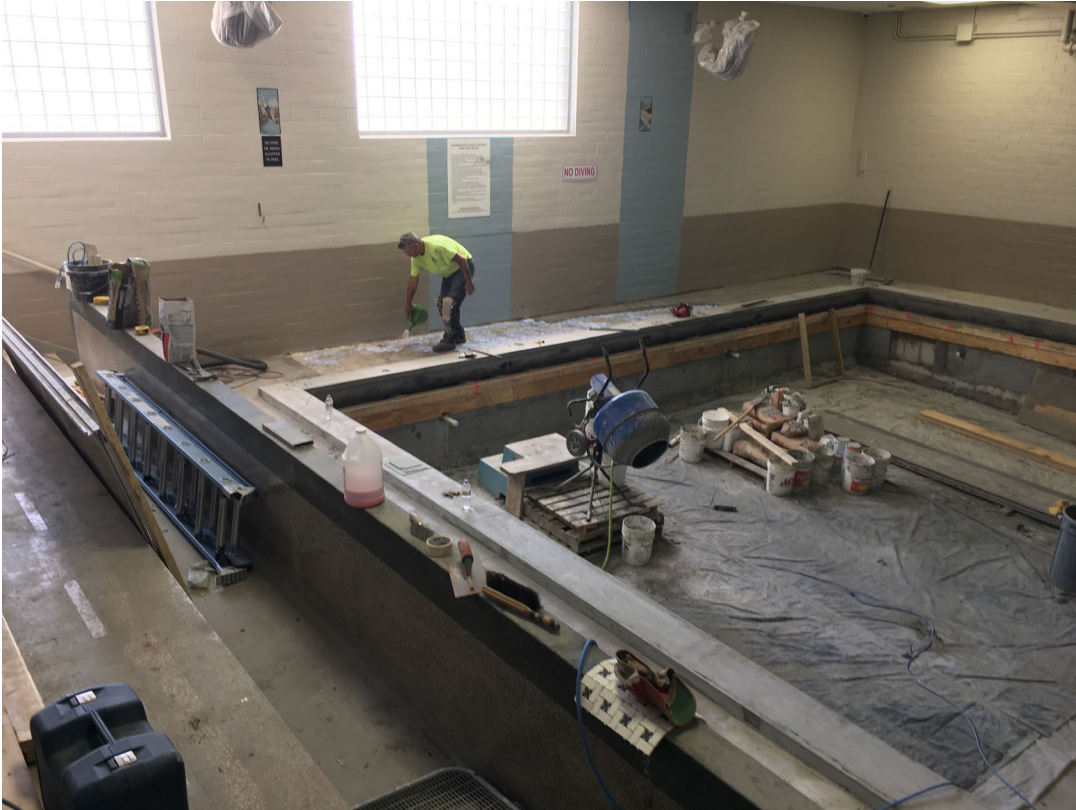
Preparations for deck epoxy flooring
