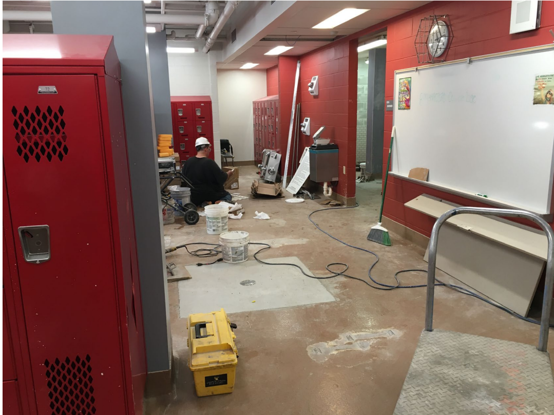
Renovations in girl's locker room
