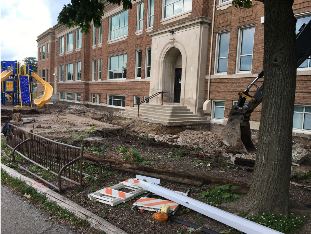
Installation of drain tile
