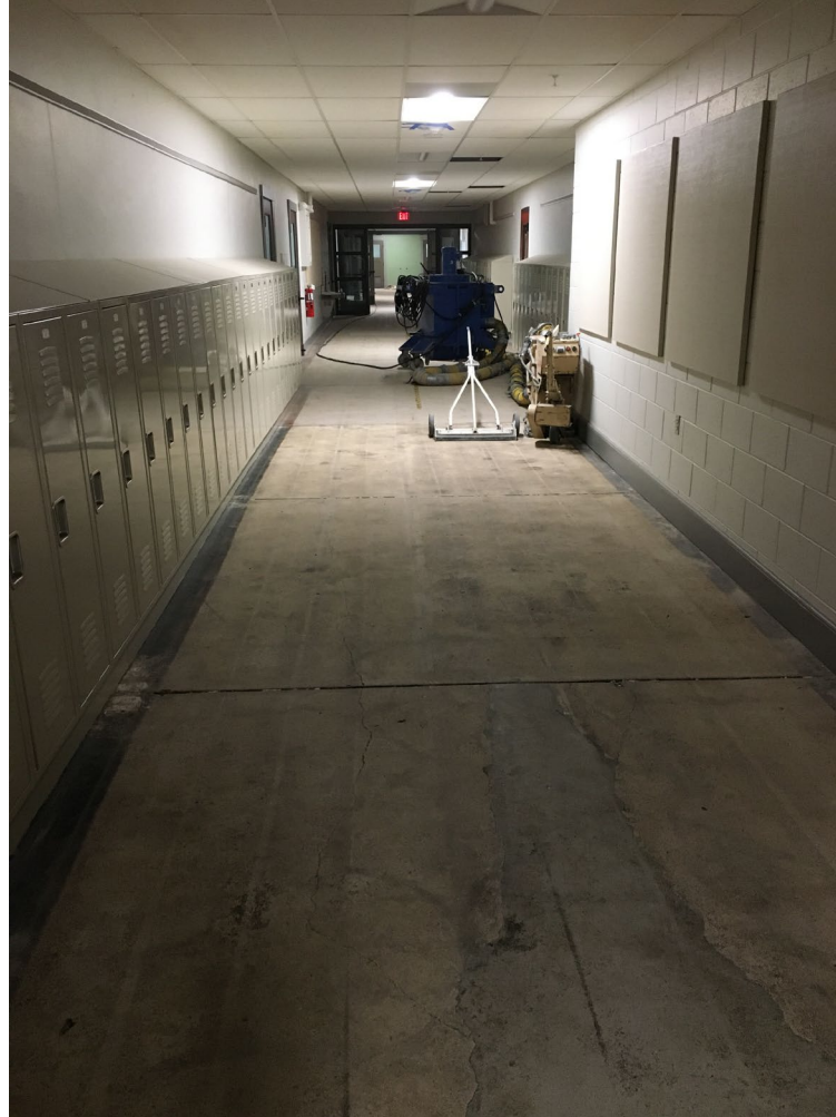
Preparations for lower-level corridor epoxy flooring
