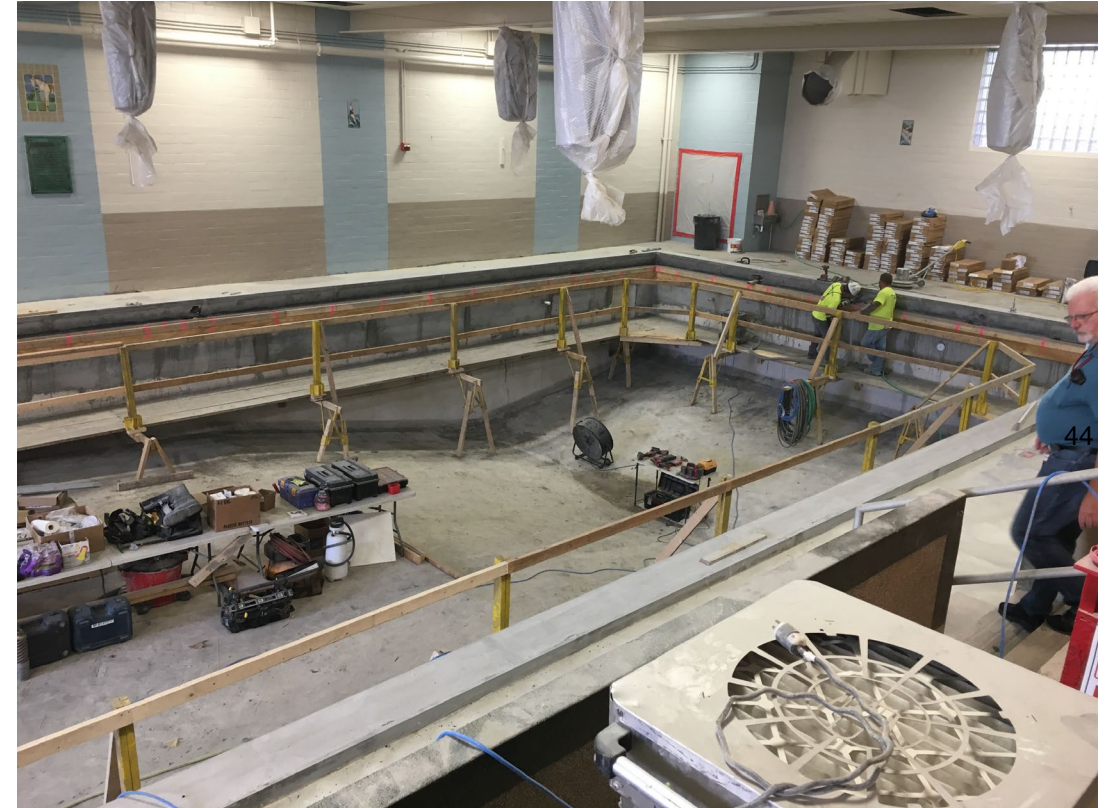
Preparations for plaster finish
