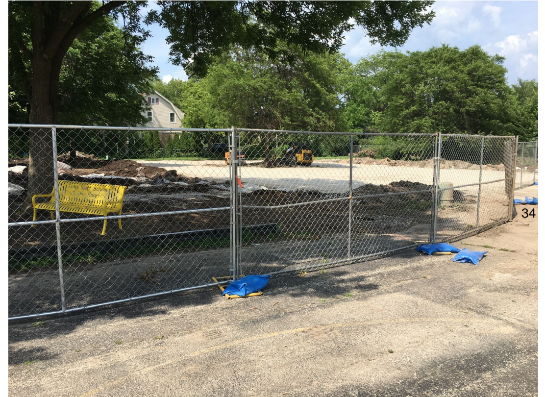
North playground work has begun
