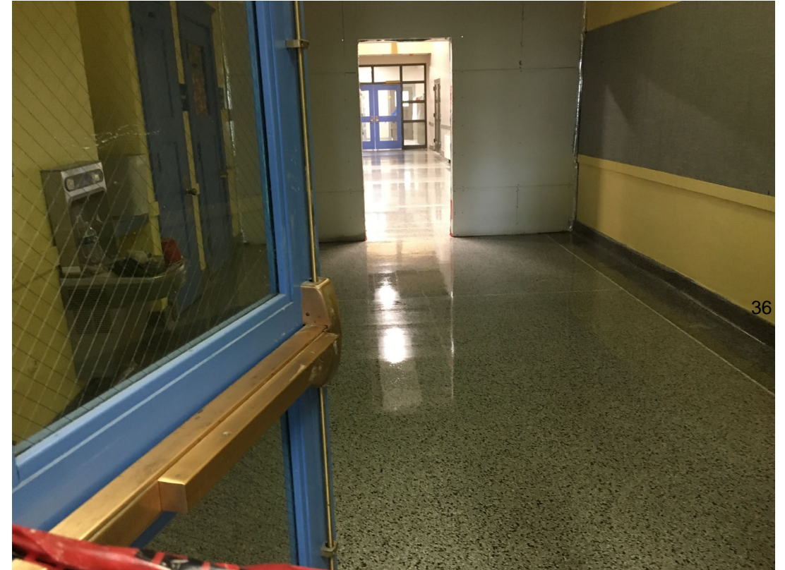
Refurbished terrazzo floors
