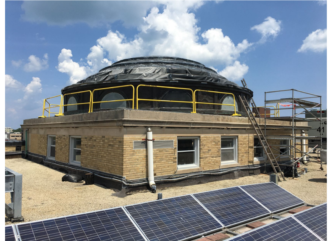
Copper Done Exterior
