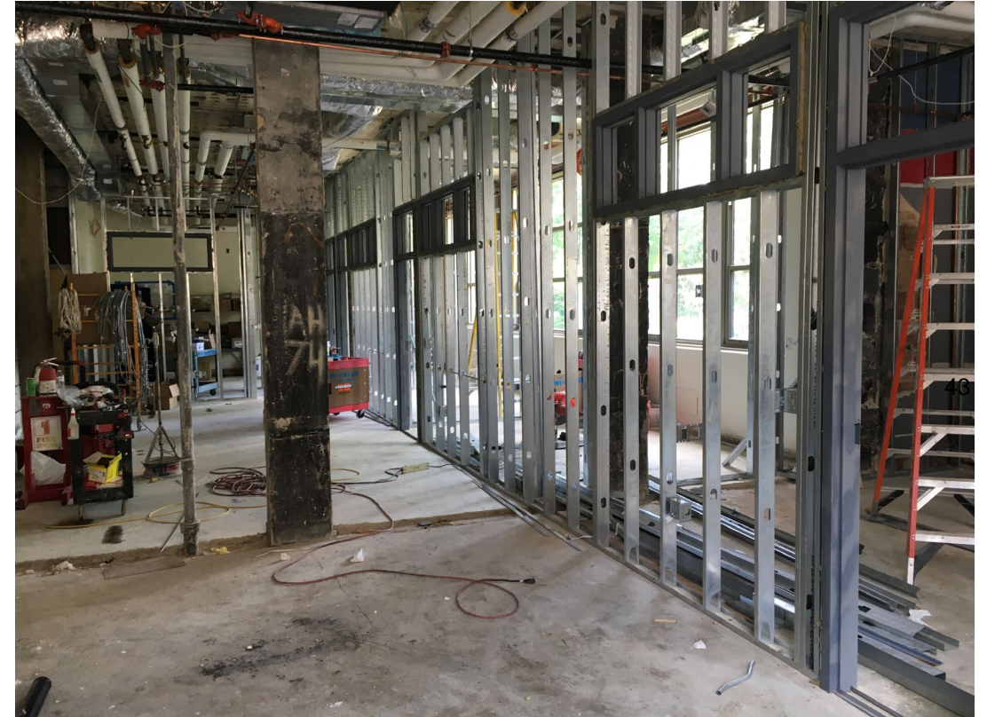
Business services office renovation
