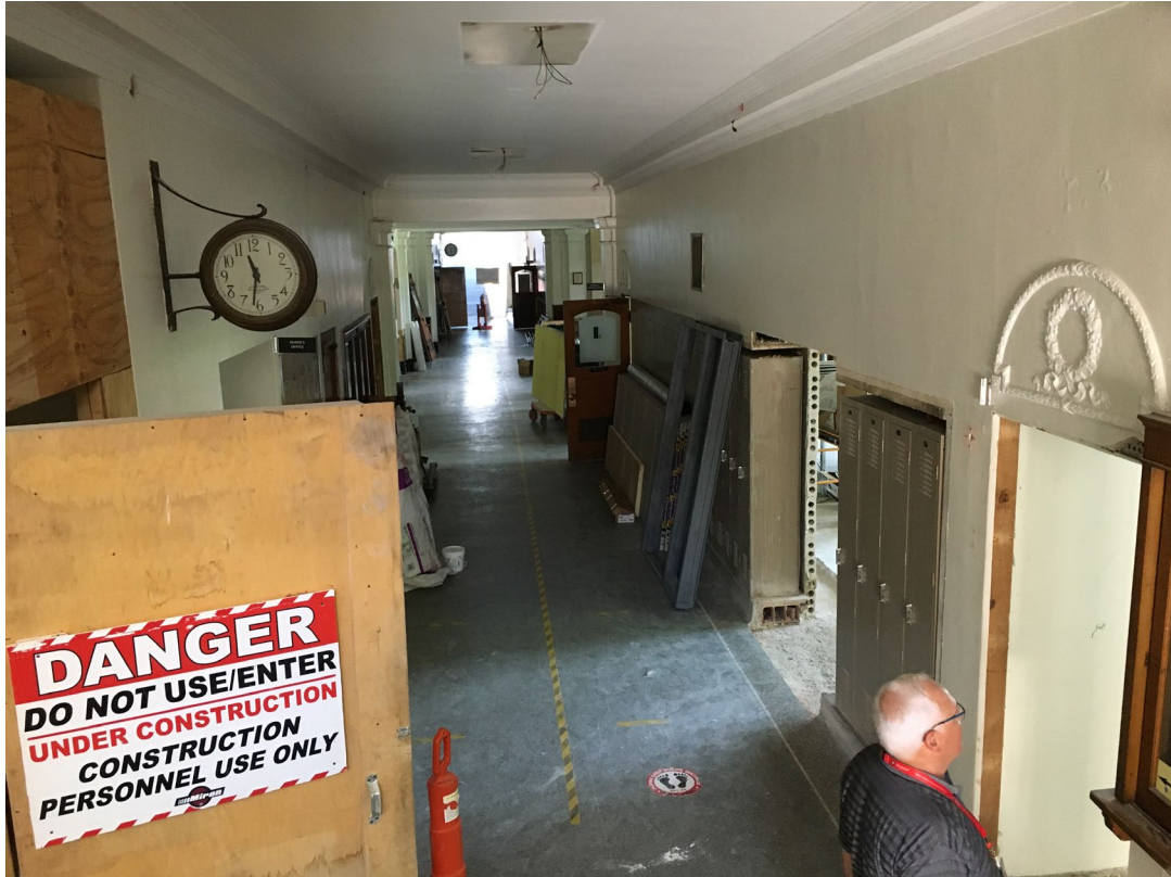
1 st floor corridor
