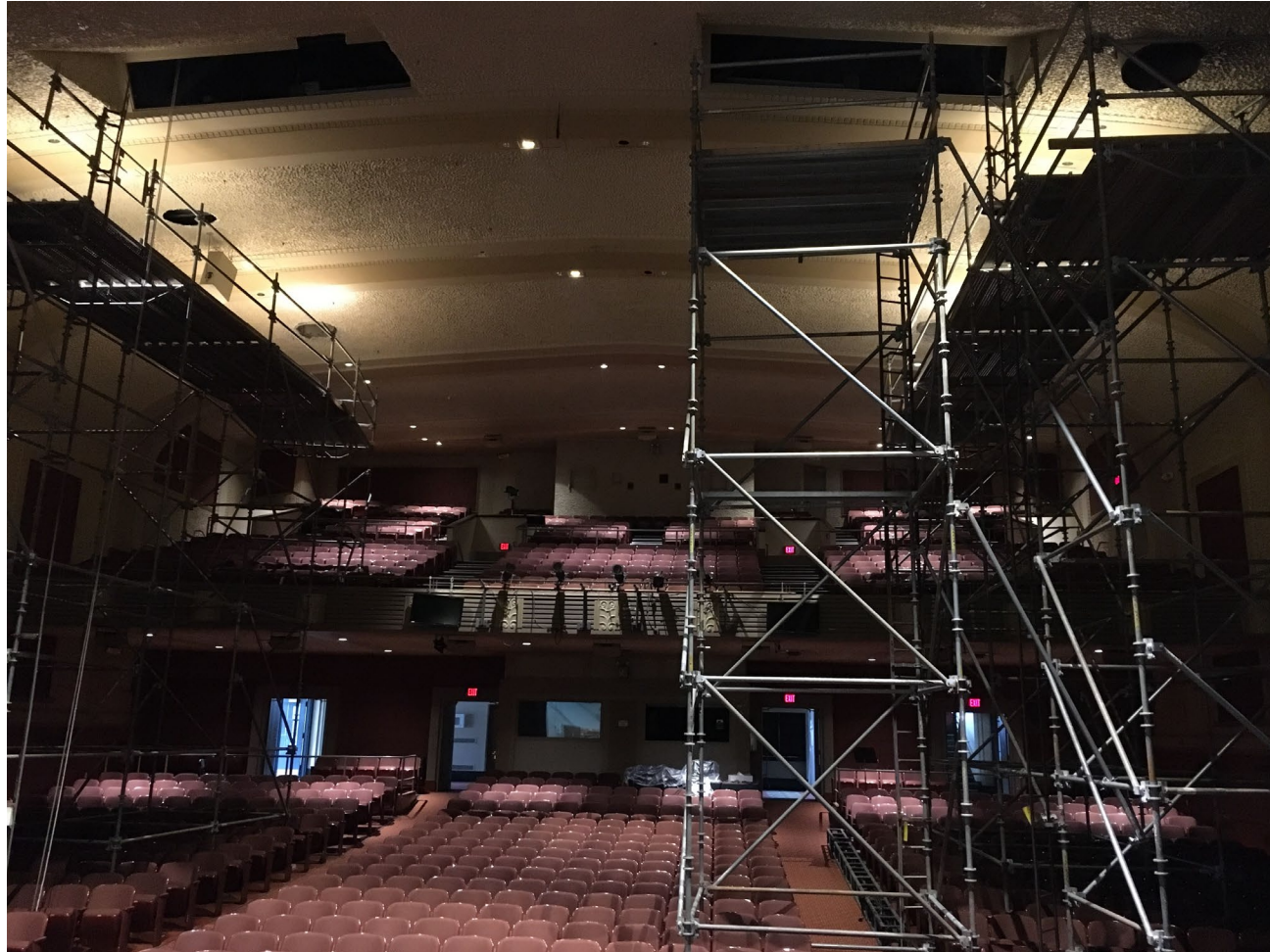
Lighting and HVAC work in theater
