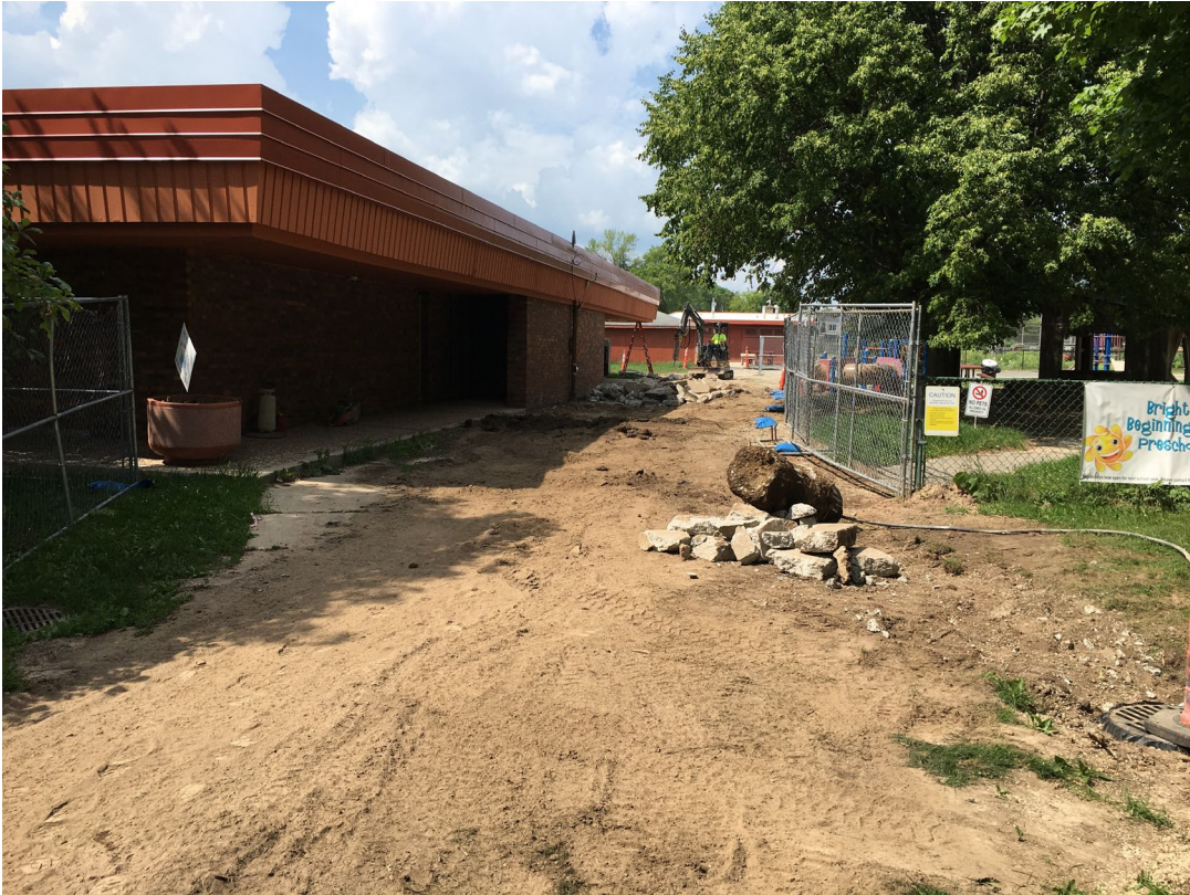
EEC concrete replacement
