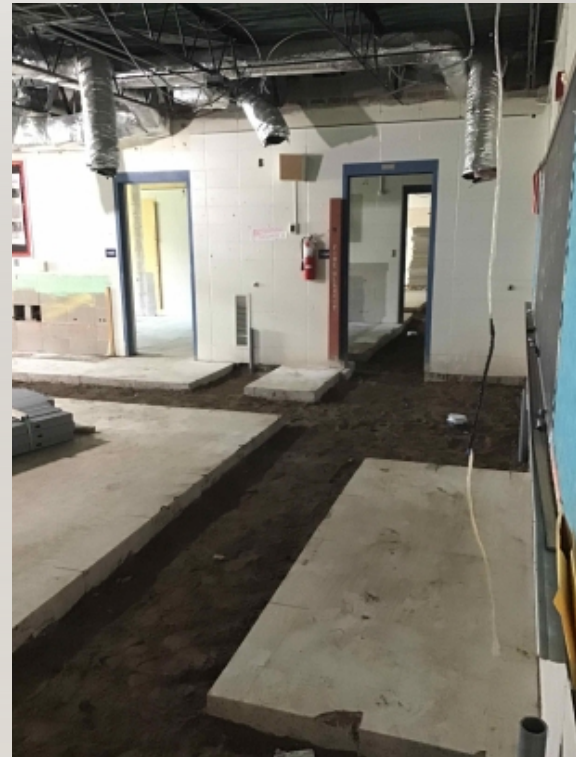
Area E Underground Plumbing
