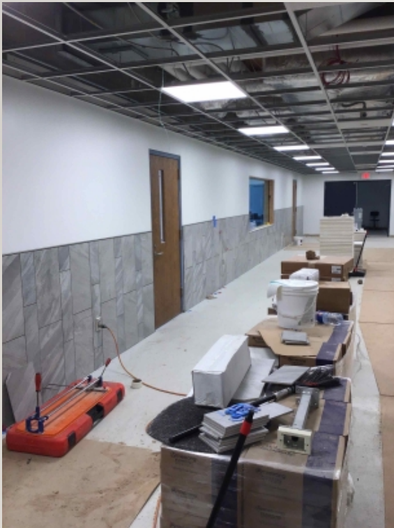
Area D Wall Tile
