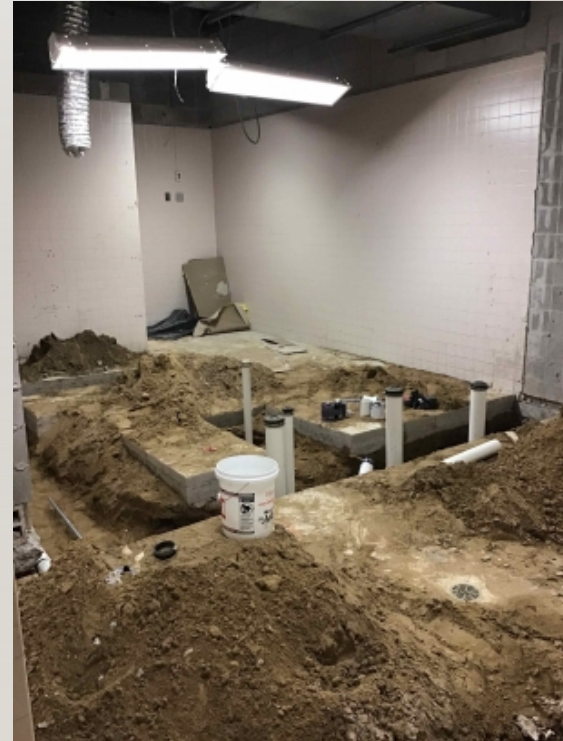
CCES Area C Restroom Demo
