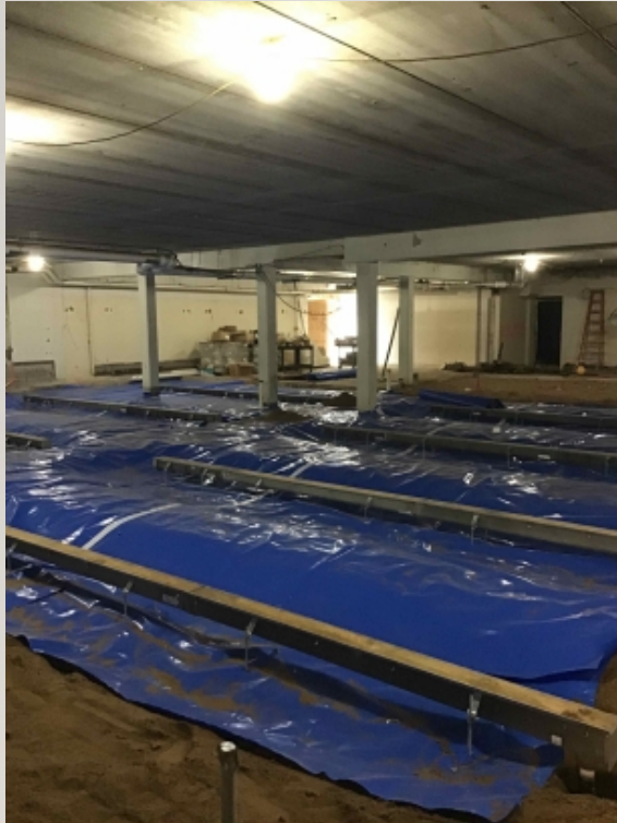
Area A Locker Room Concrete Prep
