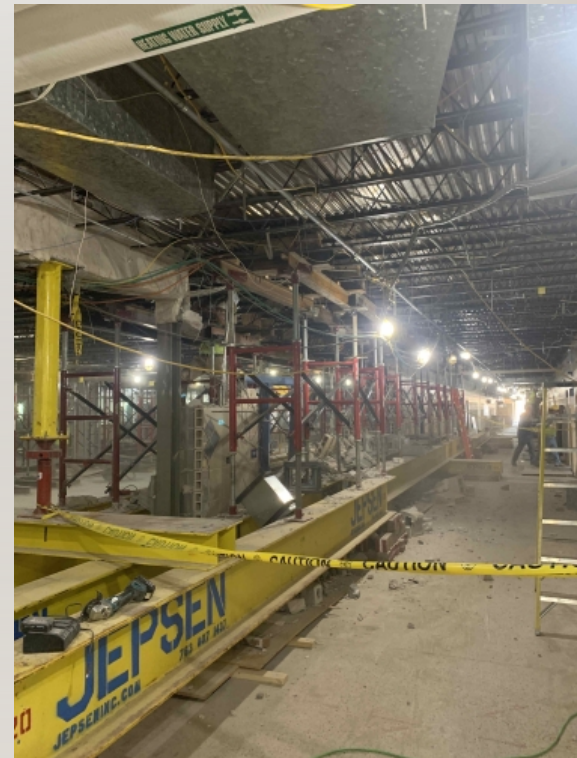
Area C Hallway Shoring
