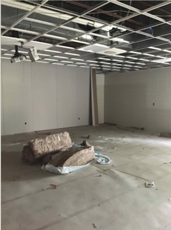
CCES SPED Area D Drywall
