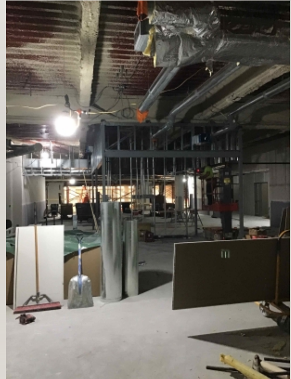
Area J Media Center Framing
