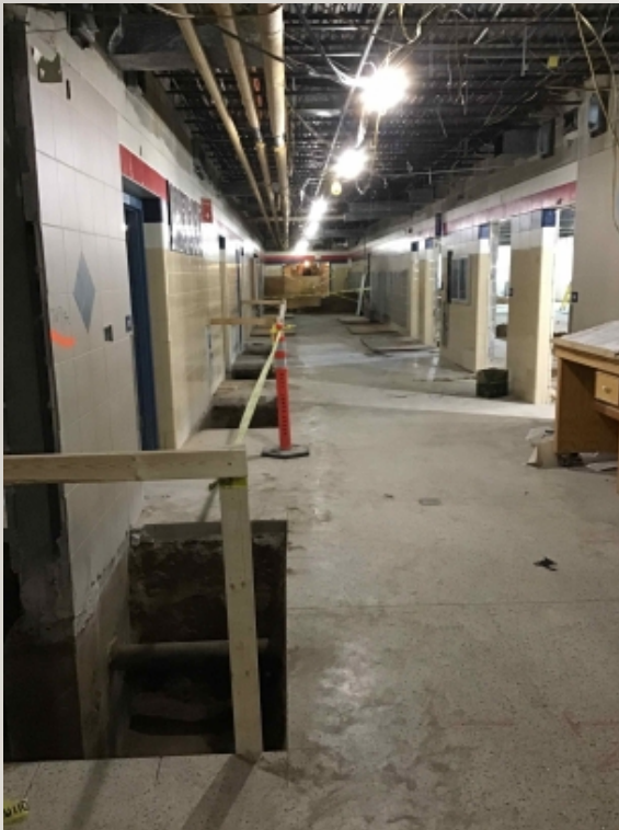
Area C Footing Prep
