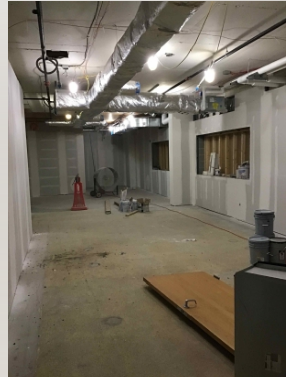
Area B Fitness Drywall Install
