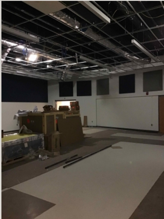
Area F Choir Room Ceiling and Wall Panels
