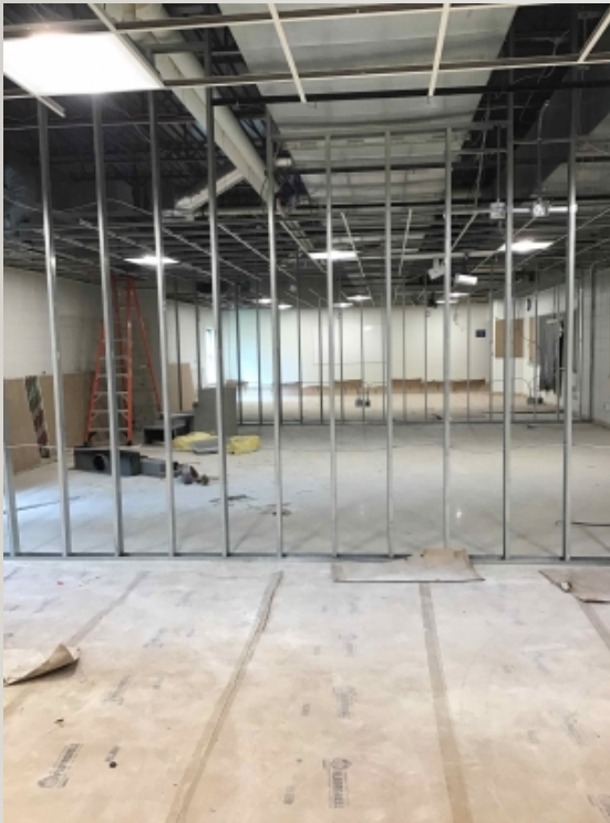
CCES Area A Wall Framing
