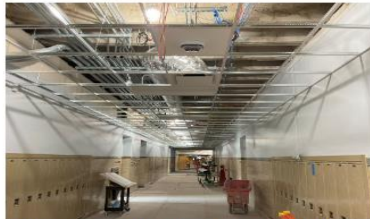
Ductwork & Ceiling Grid Installation (7/19)
