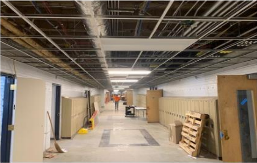
JR. ROTC During Construction – 07.24.24
