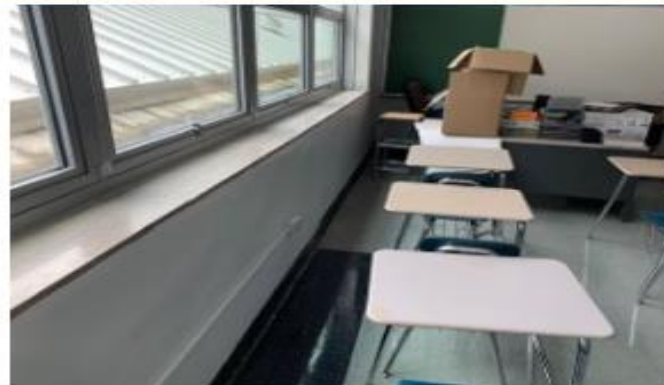
Wall and Floor Patch Back – 07.24.24
