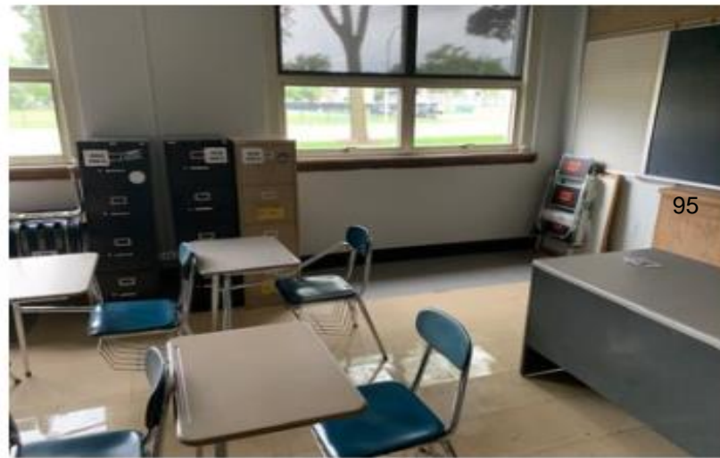
Wall and Floor Patch Back – Typical 07.24.24
