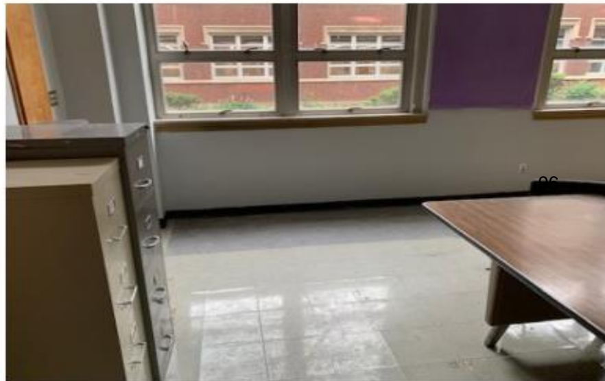
Wall and Floor Patch Back – Typical 07.24.24
