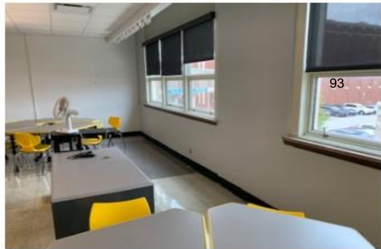
Wall and Floor Patch Back – Typical 07.24.24
