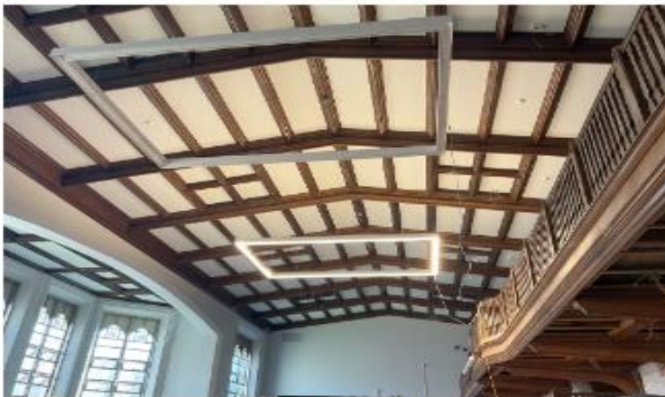
Library Lighting Installation (7/19)
