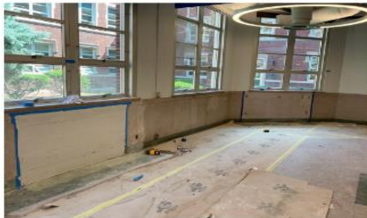
Cafeteria Terrazzo Repair (7/19)
