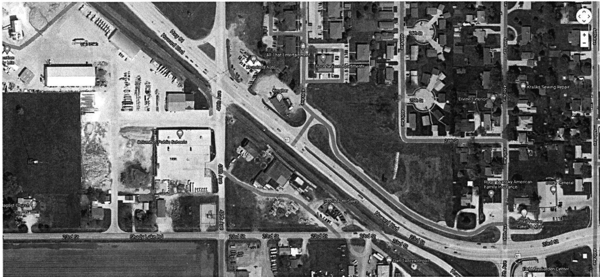
Howard Blvd. corridor affected by new fire station. Intersection lights at 45 th Ave and 48 th Ave will be controlled.
