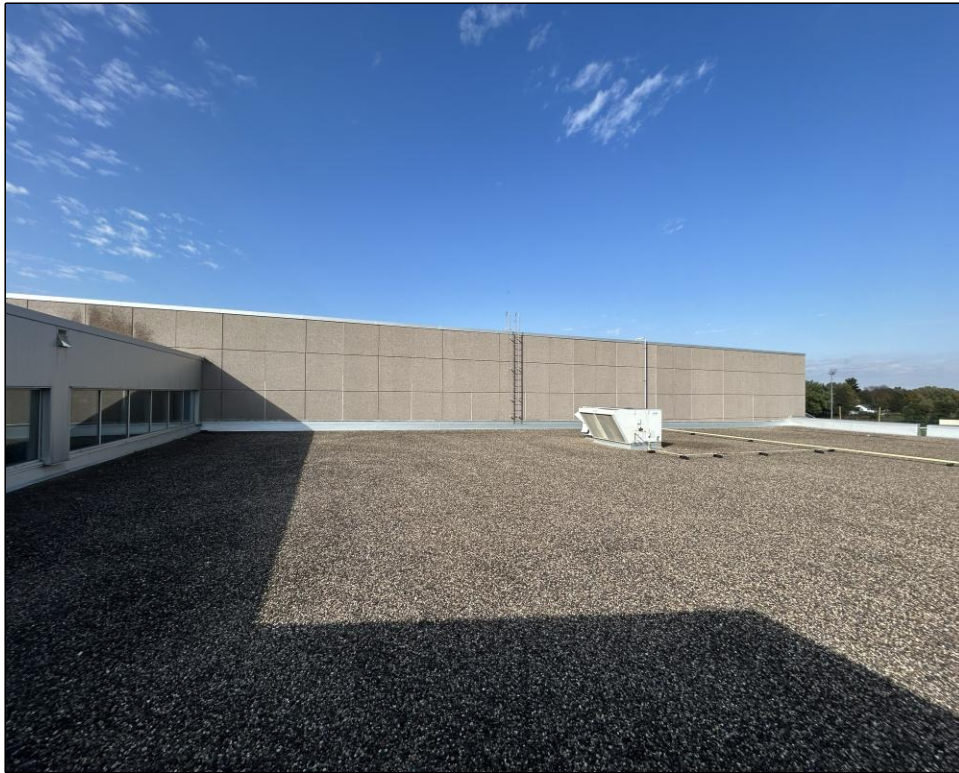
Control joint replacement overview photo.
