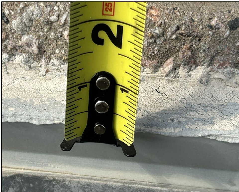
Horizontal sealant joint width.
