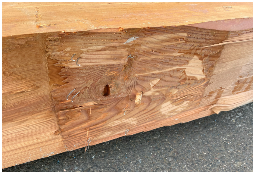
Figure 5 – Failed Scarf Joint
