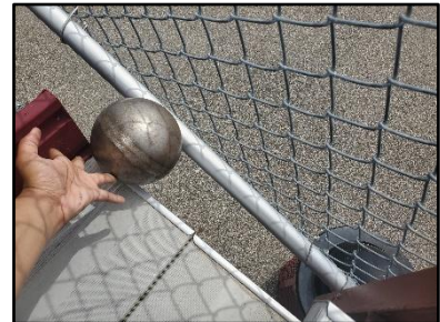
Proper guardrail gap closure.
