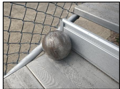
Proper guardrail gap closure.
