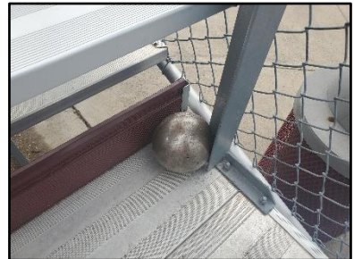
Proper guardrail gap closure.
