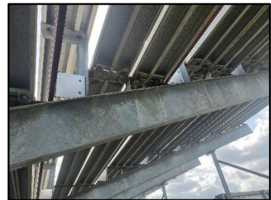
Galvanized I-beam frame design.
