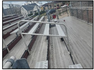
Mid aisle handrail.
