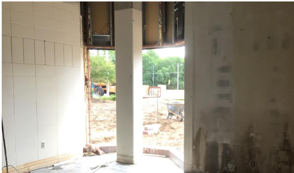
Bay Window Demolition
