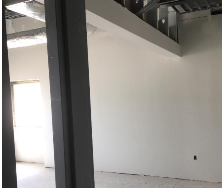
North Addition Progress
