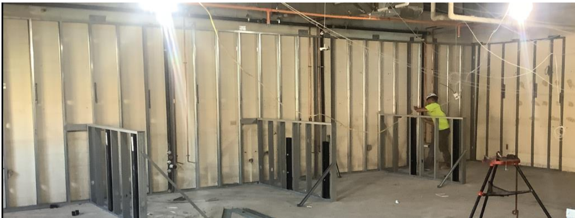
HS FACS Lab Framing
