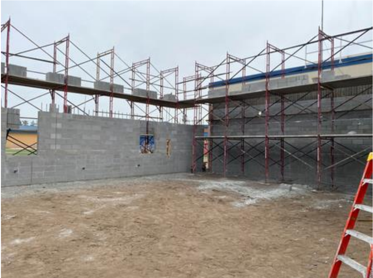
Masonry Walls around Early Childhood addition
