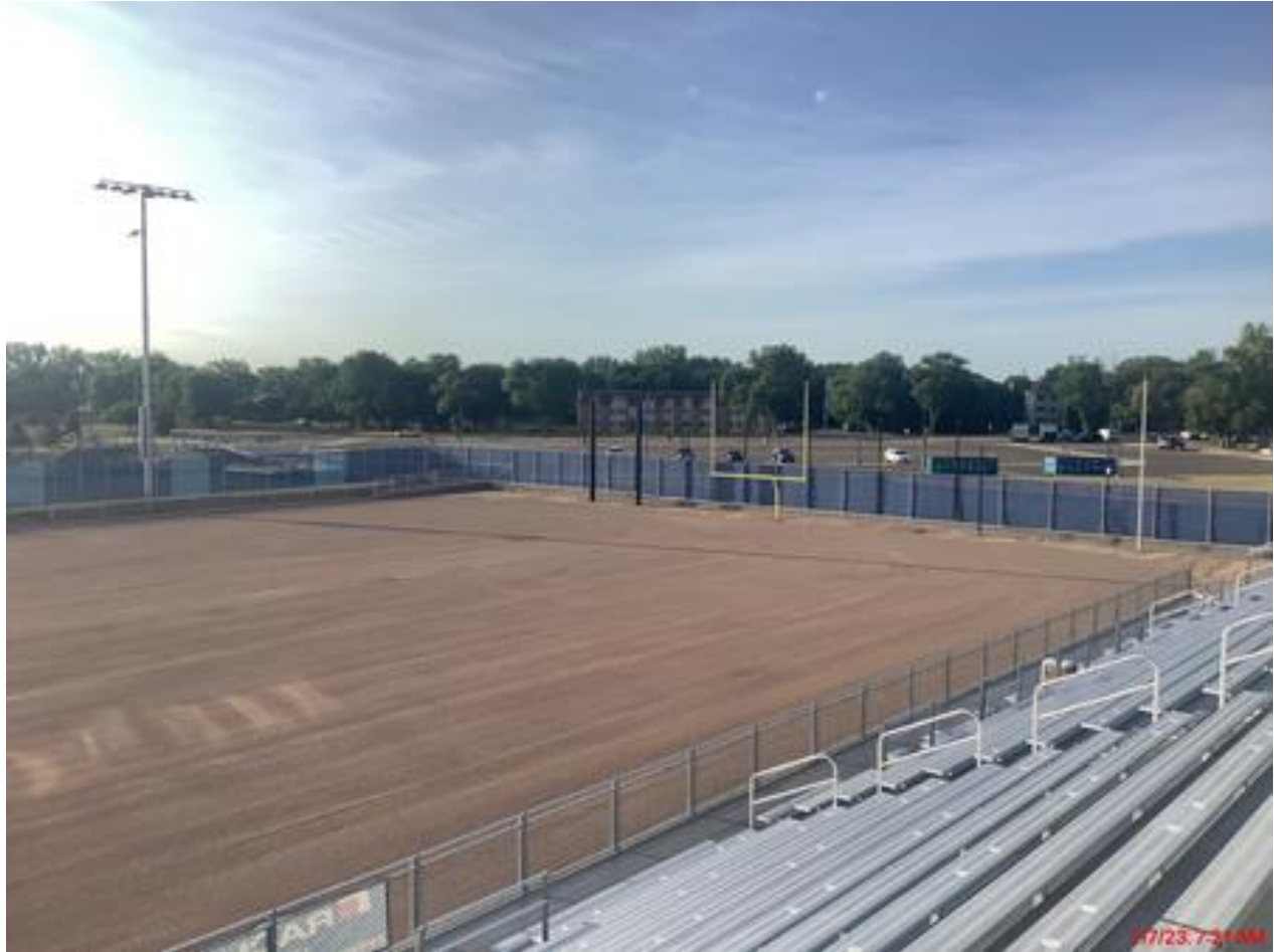
Fencing installed, scoreboard and timeclock posts installed
