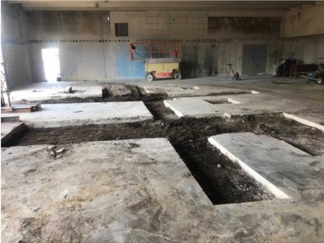
Concrete removal and underground plumbing ongoing throughout Early Childhood
