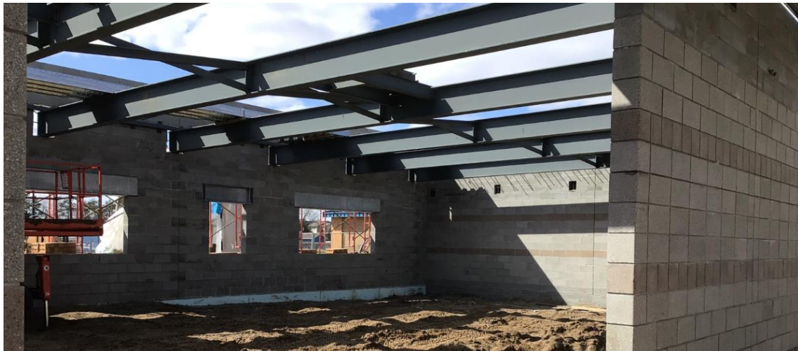
South Addition ready for decking
