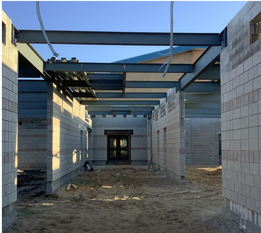
South Addition corridor
