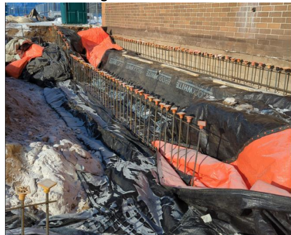
Footings and Foundation
