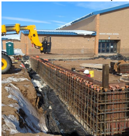
Foundation Wall Prep
