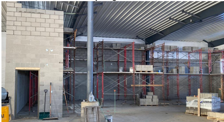
Wash Bay Progress
