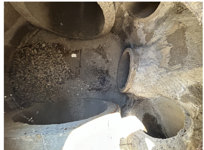
③ NON-STANDARD DRAINAGE STRUCTURE
