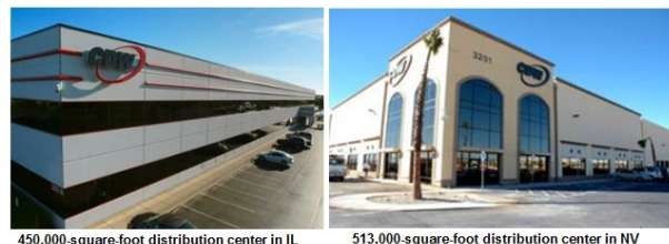
450,000-square-foot distribution center in IL
