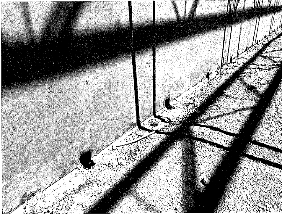
Precast connections
