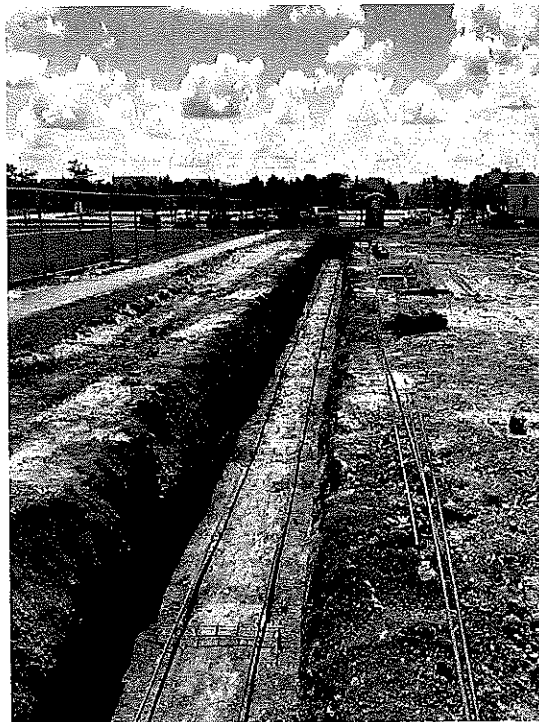
excavations for trench footings for new gym
