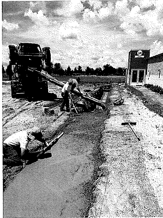
concrete placement for trench footings for new gym footings
