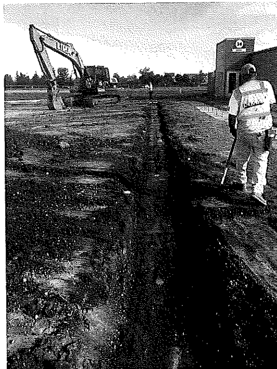
Looking north on thicken slab area
