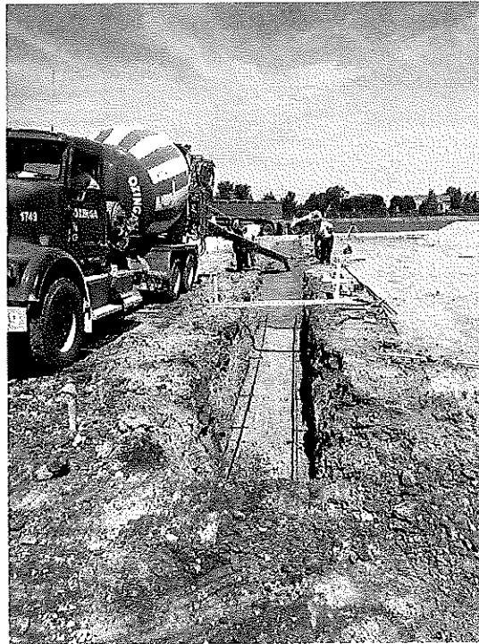
Concrete placement for trench footing for new gyl looking north on west footing
