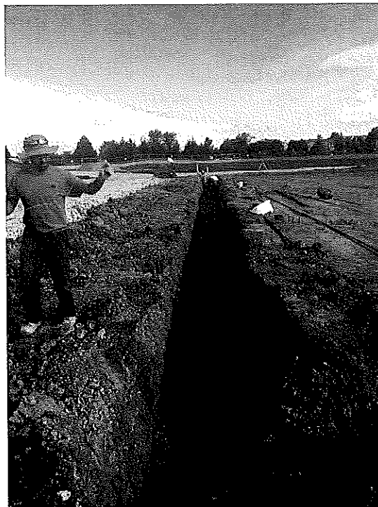
looking north on west trench footing
