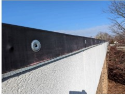
EPDM fastened to the cleat
