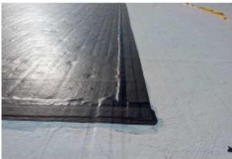
6" cured cover strip installed along the edge
