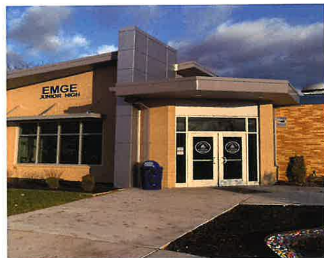
Veregy assisted with the new front entrance at Emge JH, and repaved the asphalt drive and concrete sidewalk around the front entrance.
