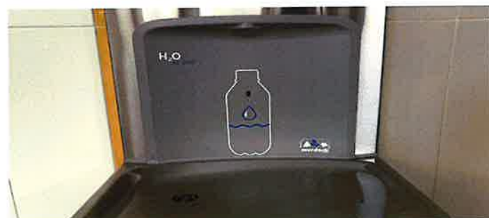
Drinking fountains were replaced with new models equipped to fill containers that did not require any hand touching, thus avoiding the spread of germs.
