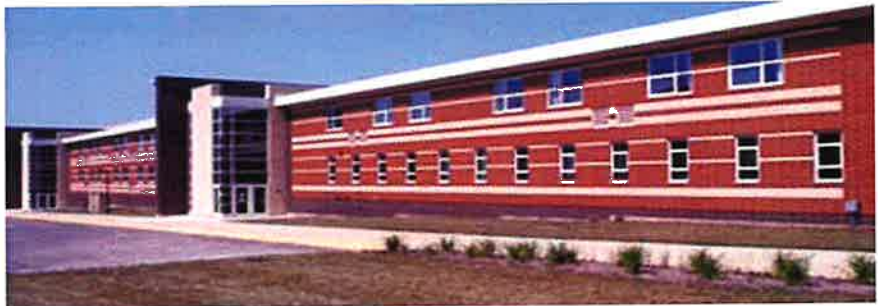
Veregy designed renovations at McHenry West High School, installing an energy efficient HVAC system, geothermal loop system, and building automation system, saving over $255,000 annually.
