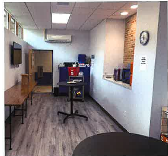
One room was converted to a STEM classroom with new HVAC, floors, walls, and ceiling with LED lighting.
