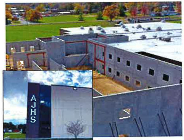
Veregy managed the construction of the new Junior High.
