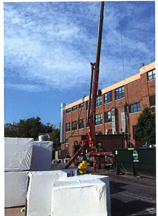
Preparing to lift new roof top HVAC units onto the roof at McHenry East High School.
