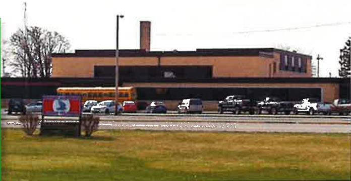
Veregy was selected to be the Energy Services Company for Heritage CUSD 8. Upgrades to bathrooms and locker rooms were completed.
