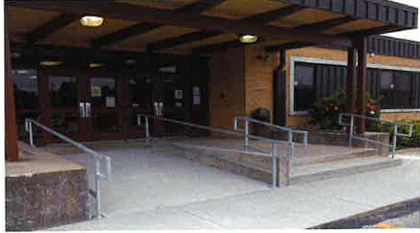
Veregy installed new hand rails for ADA accessibility.
