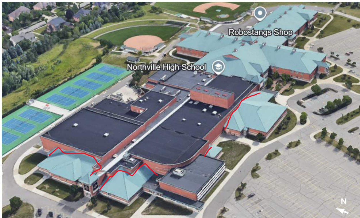
Figure 2. Annotated aerial view of the school identifying the extent of reported water infiltration at metal roofing to masonry interfaces (red lines).
