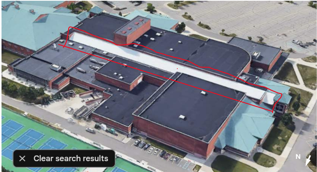
Figure 3. Annotated aerial view of school identifying the extent of reported water infiltration at the skylight (red lines).
