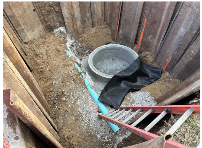
3/20: Installation of manhole base at Autumn Road.
