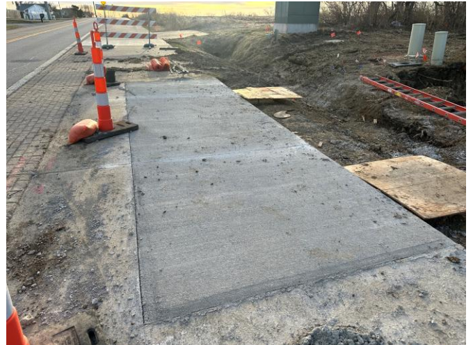
3/12: Concrete replacement for trail/sidewalk.
