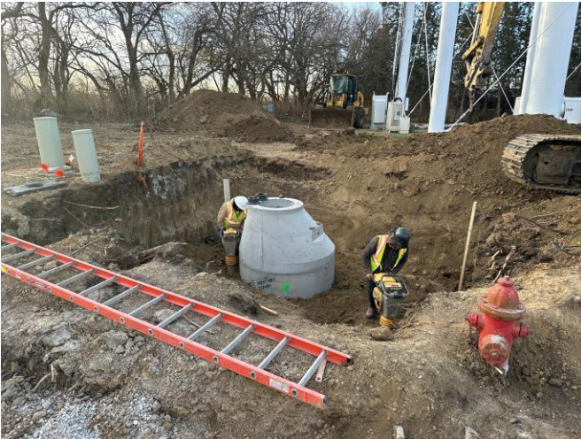
3/12: Check valve manhole top installed, backfill in progress.
