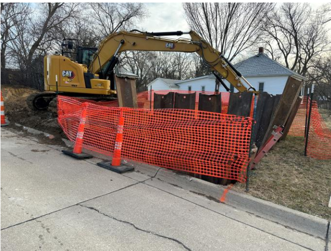
3/20: Mobilization to Autumn Road for check valve assembly installation.
