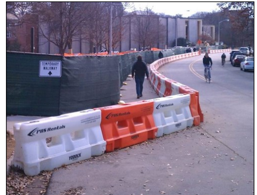
Example of a Temporary Walkway (Source: Yodock.com)
