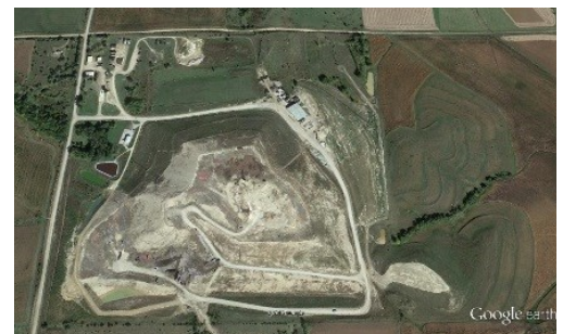
Aerial view of a Landfill, Solid Waste
