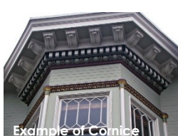
Example of Cornice
