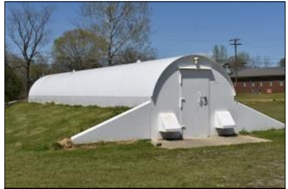
Example of a Community Storm Shelter
