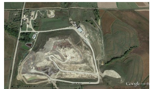
Aerial view of a Landfill, Solid Waste
