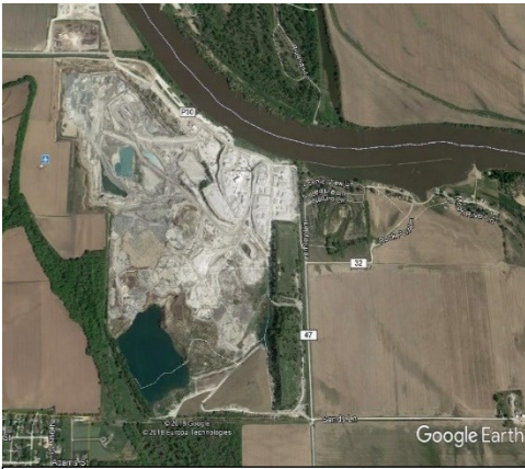
An Aerial of a Mining and Mineral Extraction Site and Quarry
