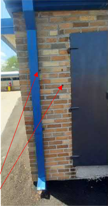
Figure 9: Remove / drill out fasteners and seal. (Option: Replace bricks with new.)
