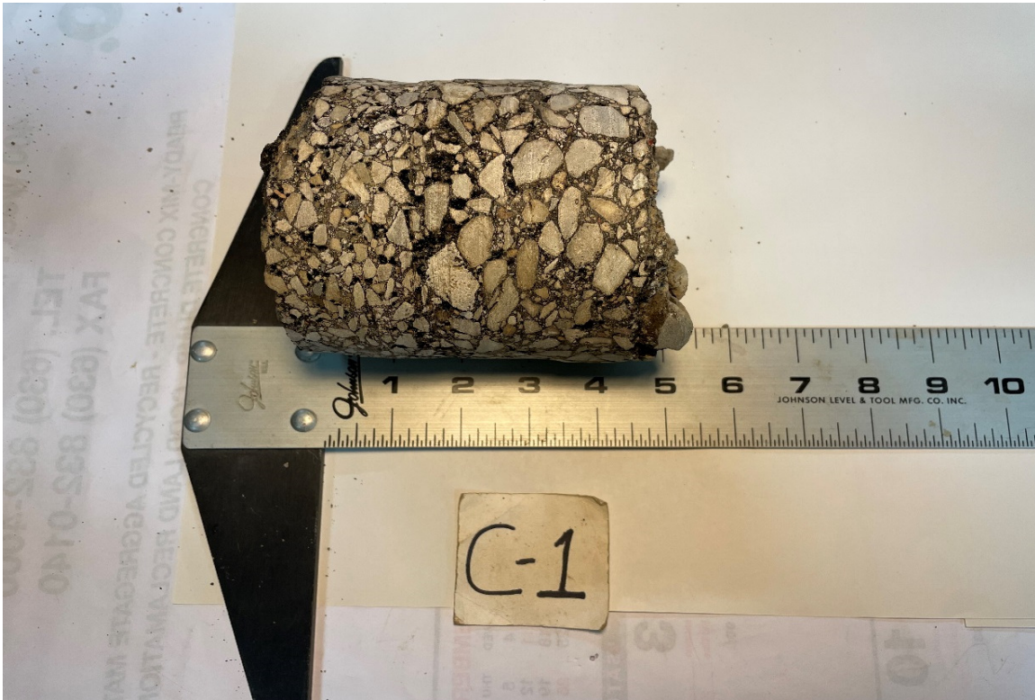
Pavement Core-1: 3925 W. Lunt Avenue
