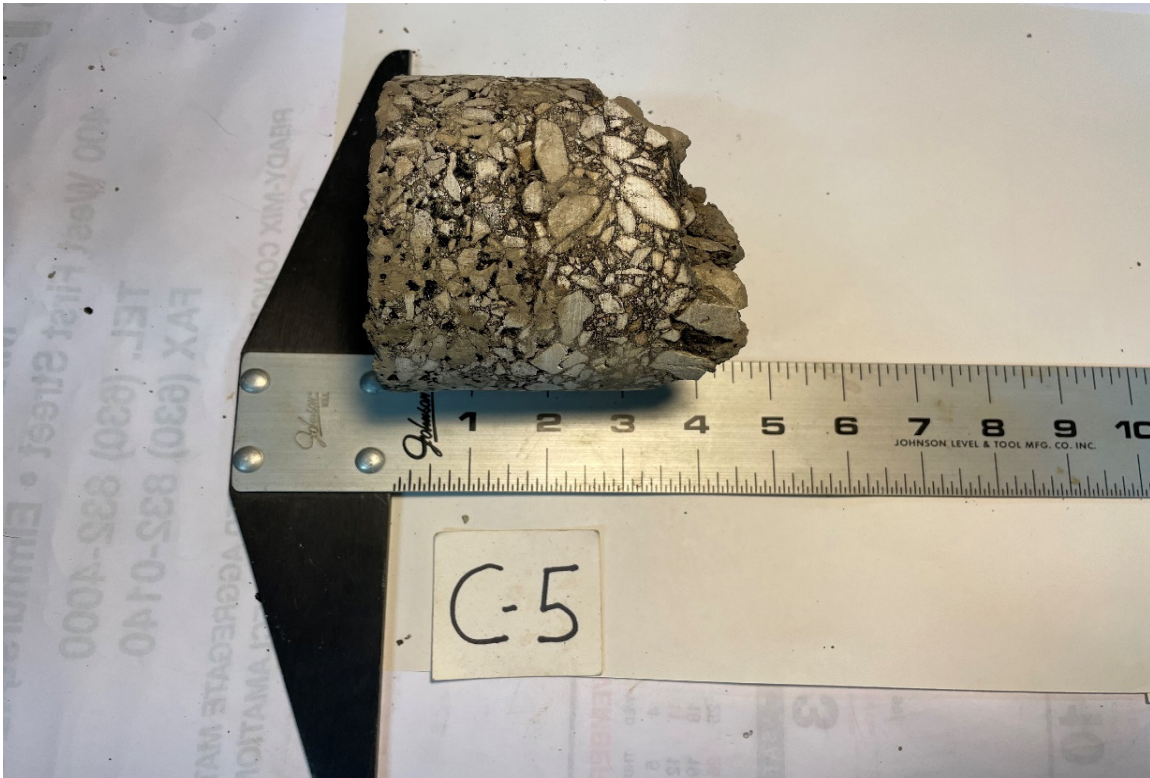
Pavement Core-5: 3925 W. Lunt Avenue
