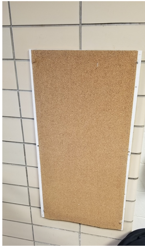
Defunct Drinking Fountain in CCDC wing
