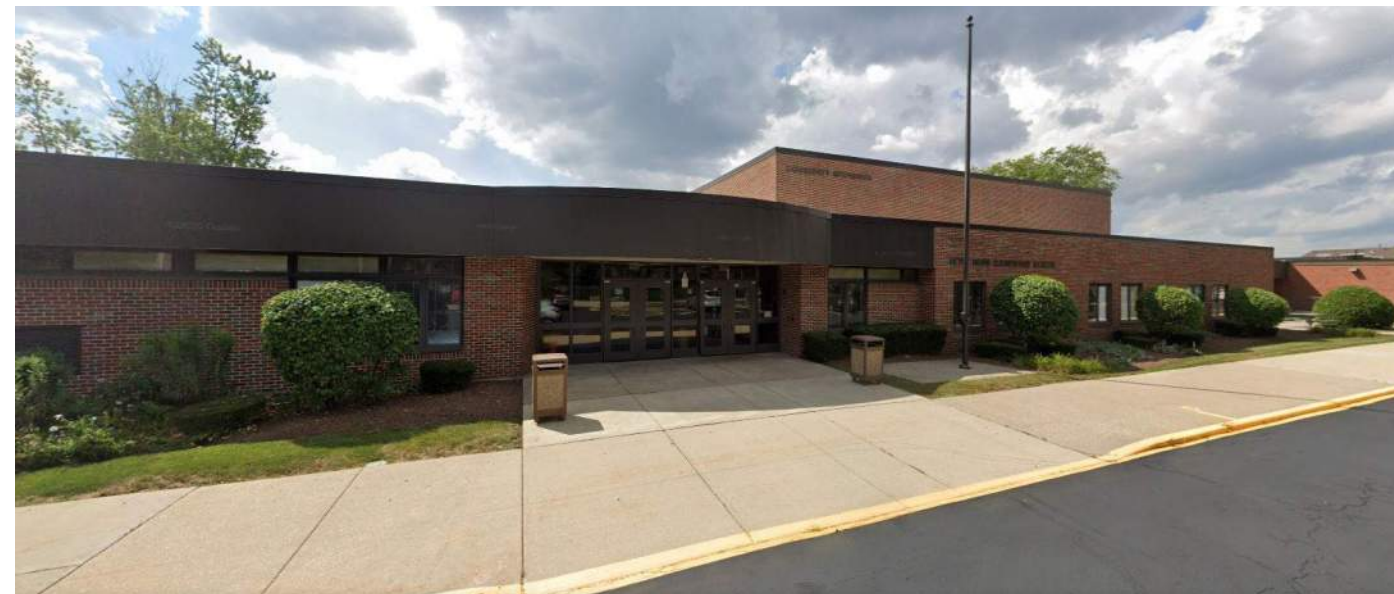
EXISTING SCHOOL ENTRANCE
