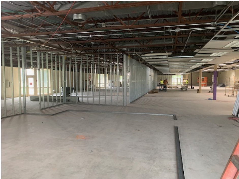
WALL FRAMING ON NORTH CLASSROOMS LOOKING E
