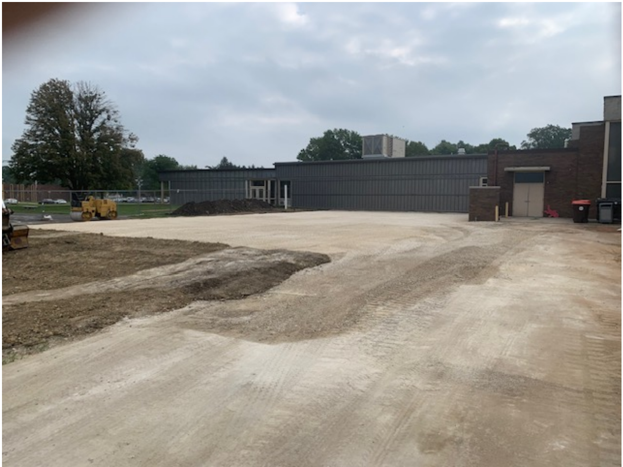
BASE AGGREGATE FOR CAFETERIA.
