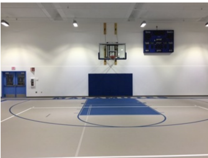
Looking at the south wall
