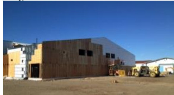
The exterior of the new gym addition taken on 9/1/2015
