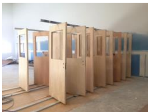
Doors being prepped for install... most frames are already in.
