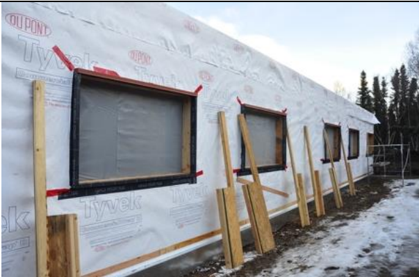
Wrapped window bucks and added metal drip flashing
