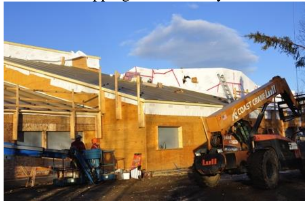
Installing roof panels
