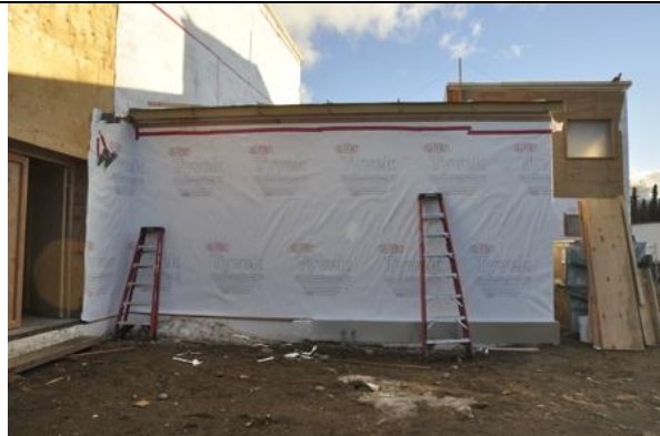
Wrapping exterior in Tyvek
