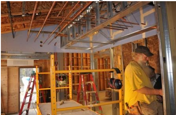
Constructing soffit outside Kindergarten Rooms
