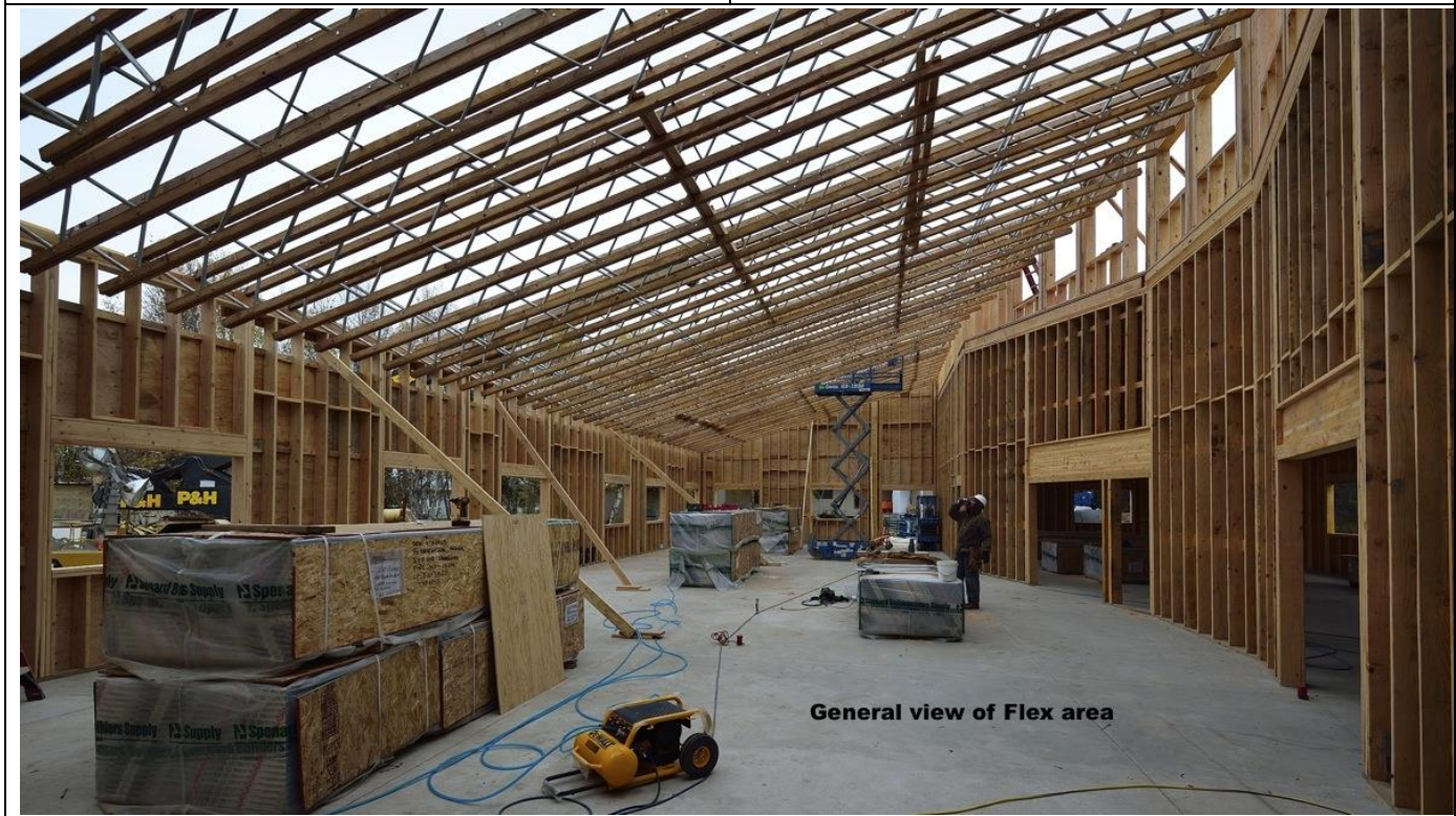
Framing interior walls – west end
