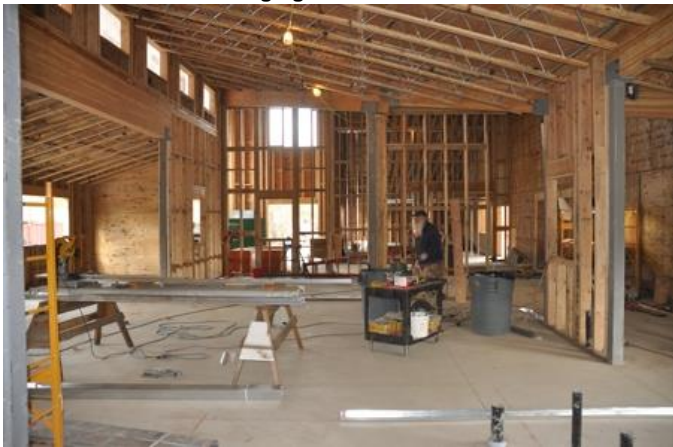
Framing interior walls – west end
