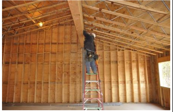
Trimming truss ends
