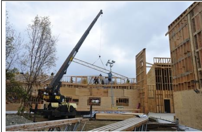
Swinging in roof trusses
