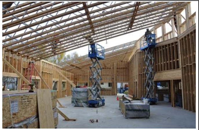
Trusses placed D.75 to G
