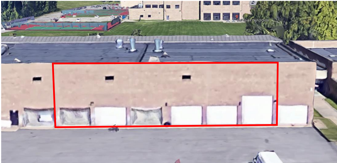
Helical Pin Work Area
