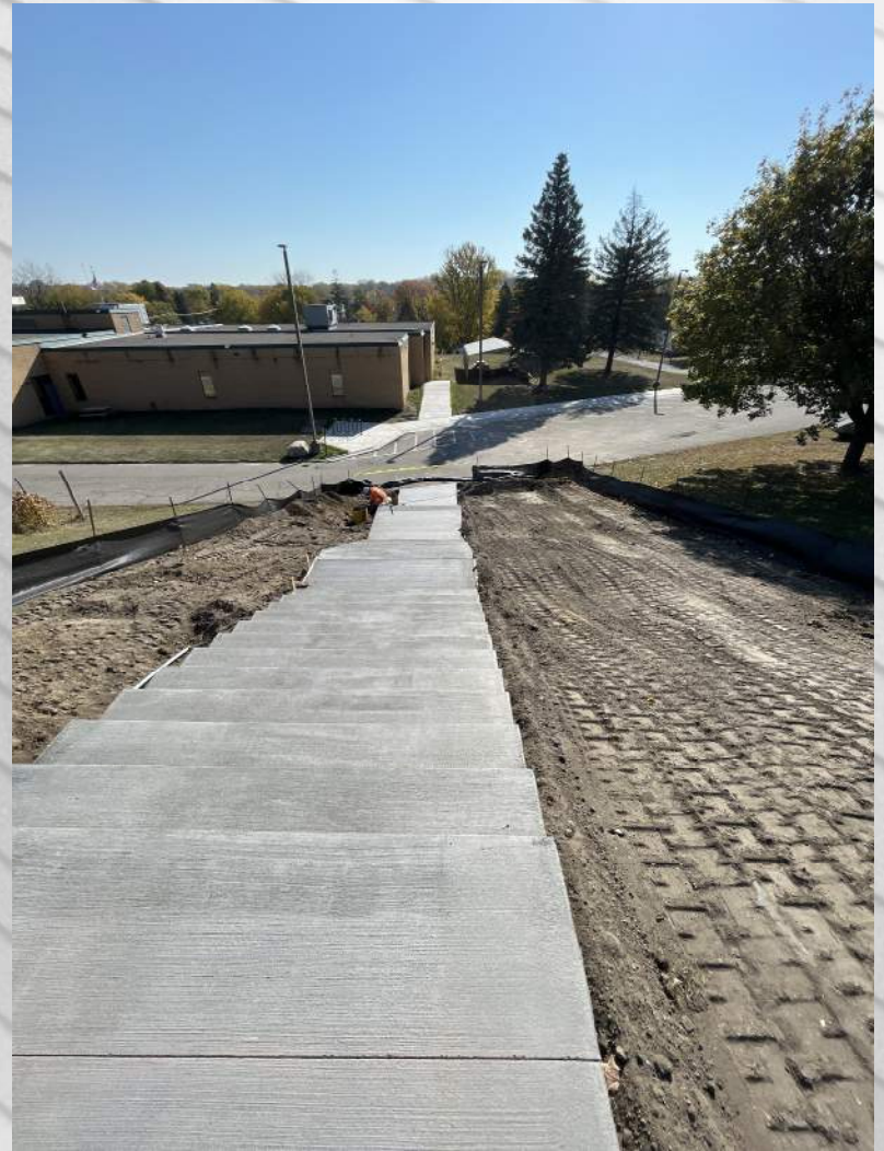
MS Stairs poured and forms removed
