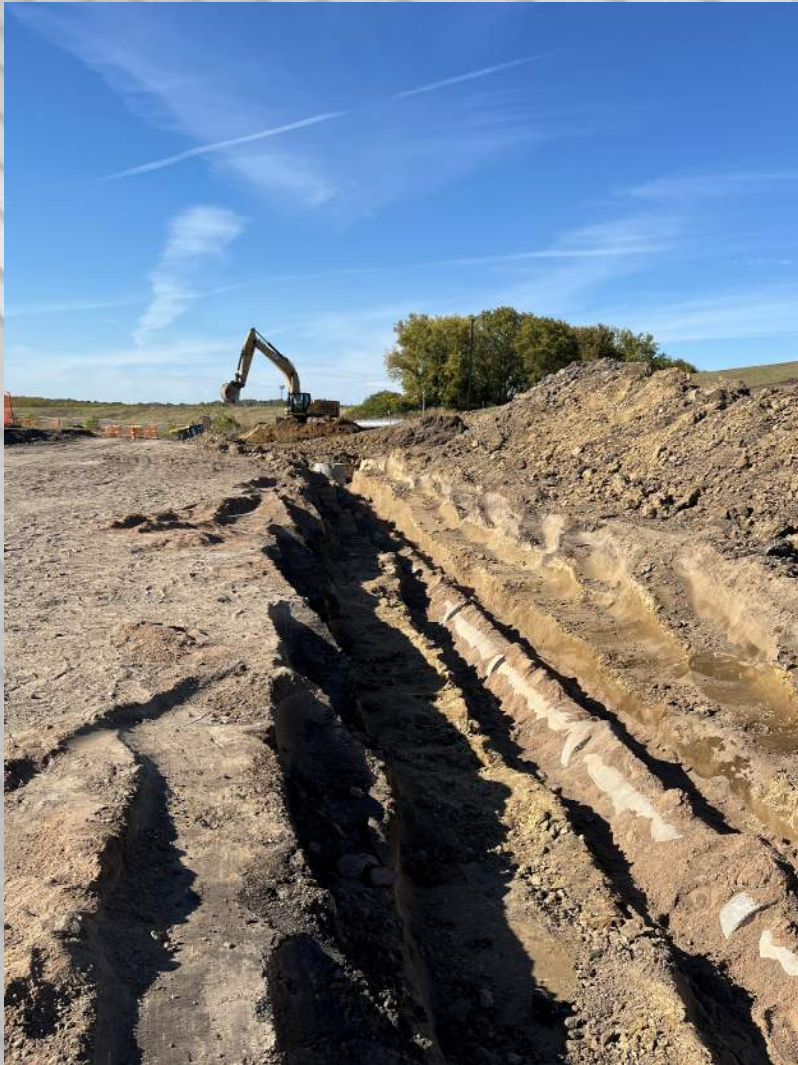
Storm sewer installation underway
