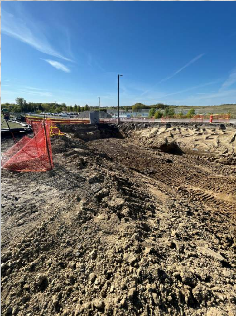
Excavations for underground storage system
